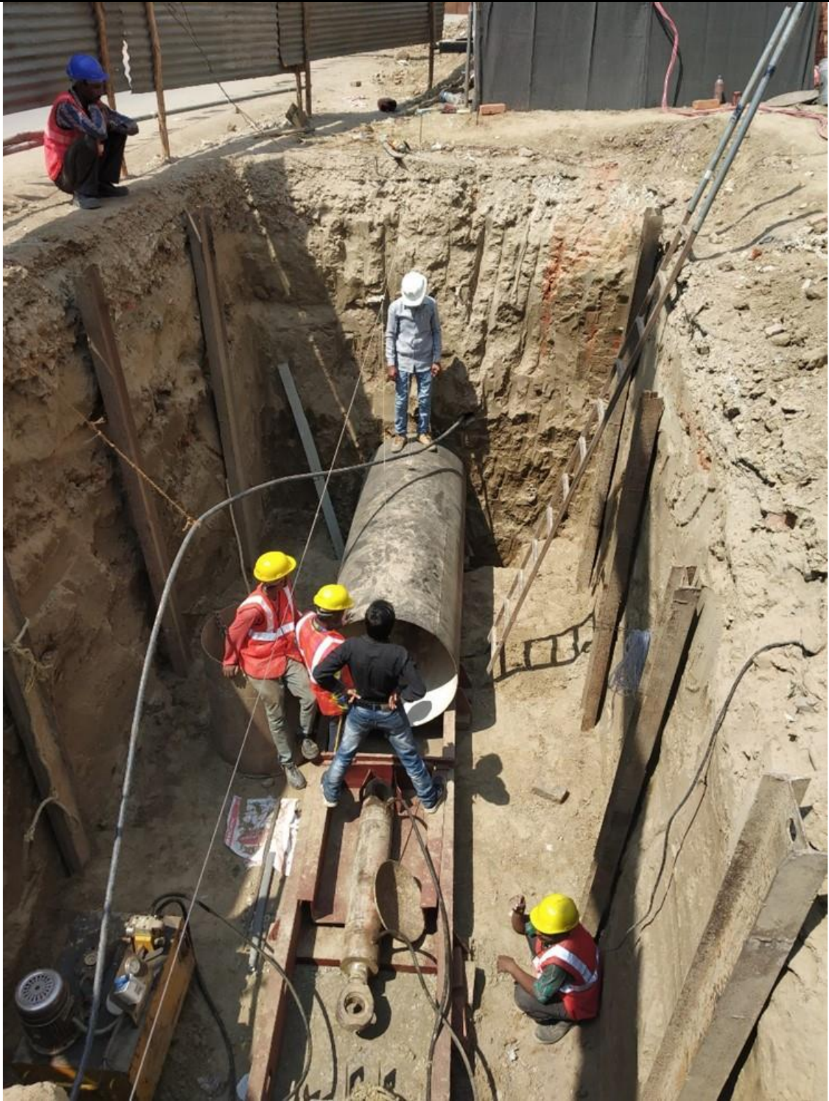
Trenchless Pipe line
