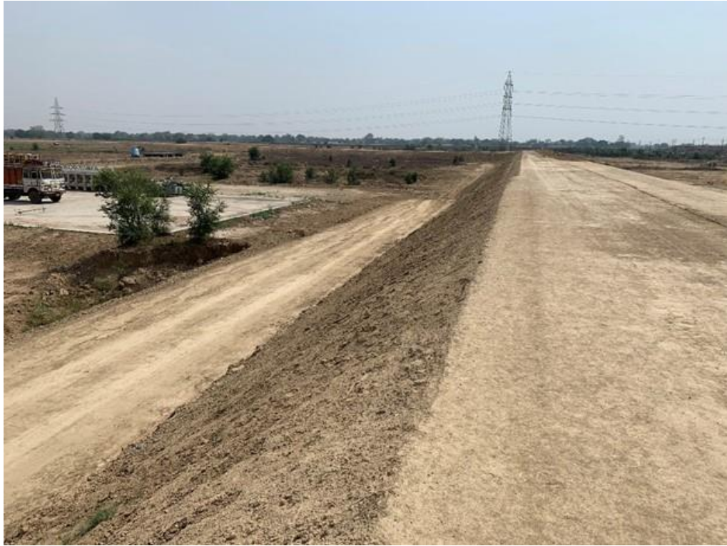
South side wall
