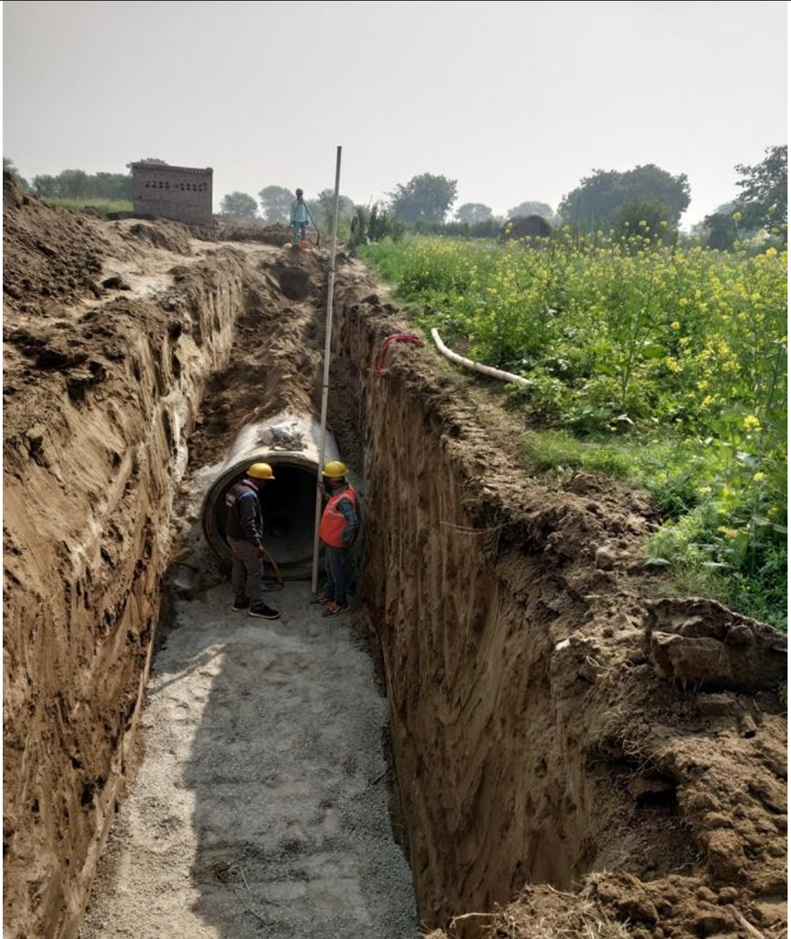
PSC Pipe laying
