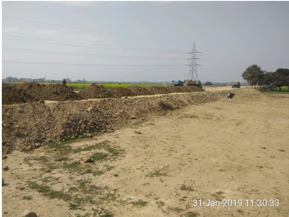
South side wall
