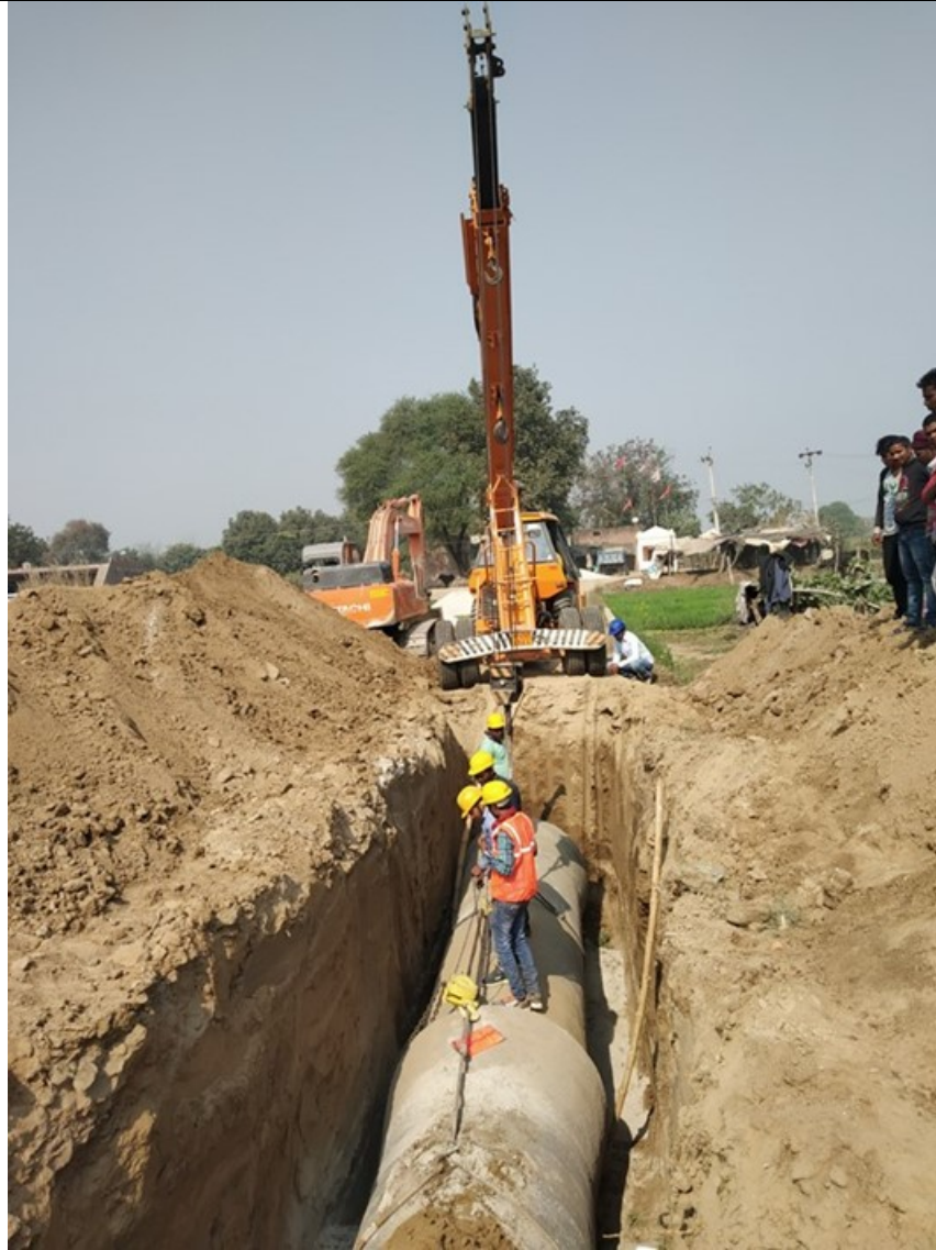
PSC Pipe laying
