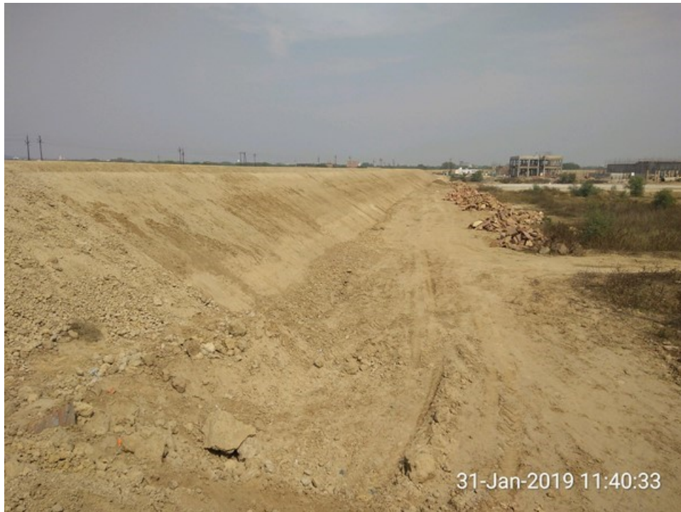
West side wall
