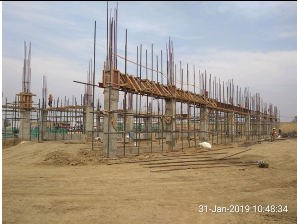
Tie beam level
