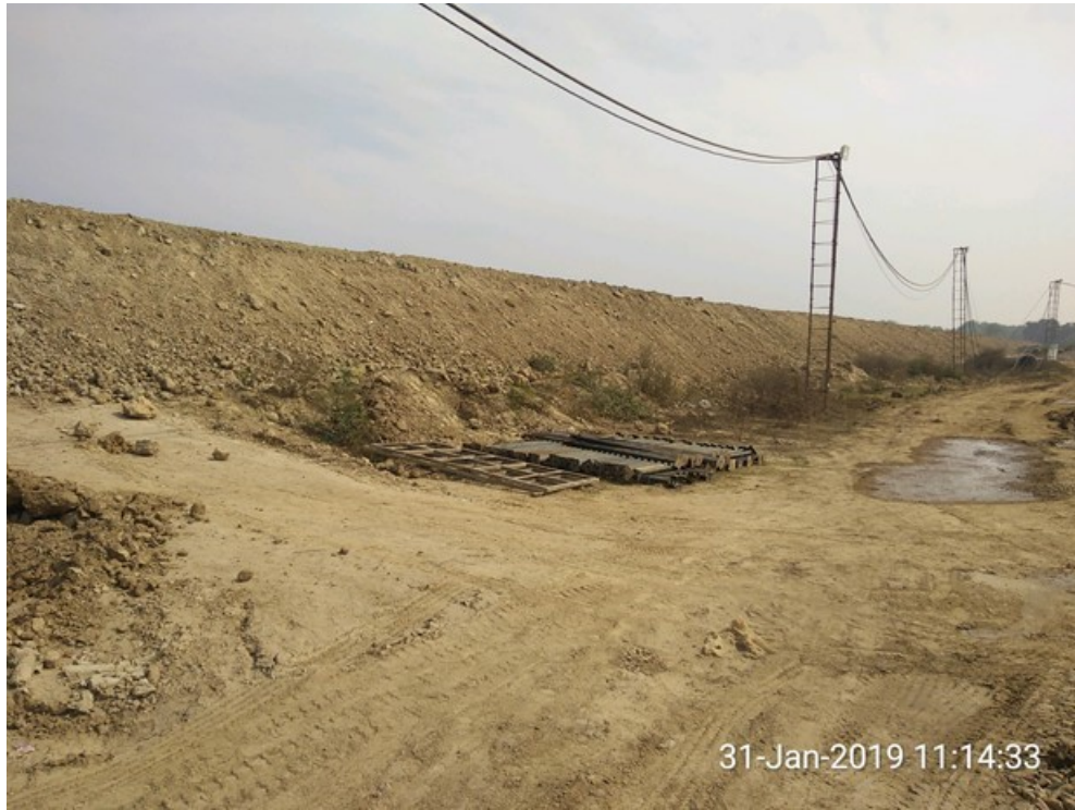
North side wall
