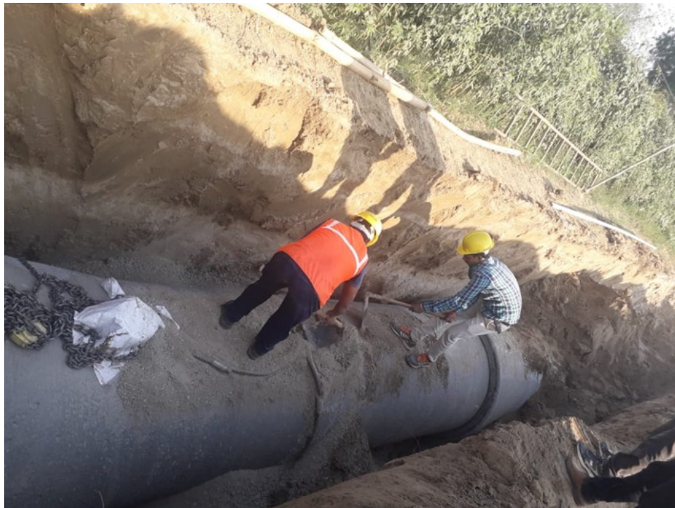
PSC Pipe laying
