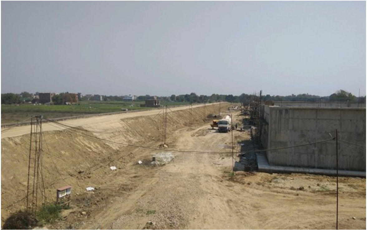
North side wall
