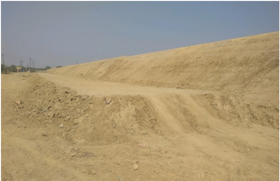
West side wall
