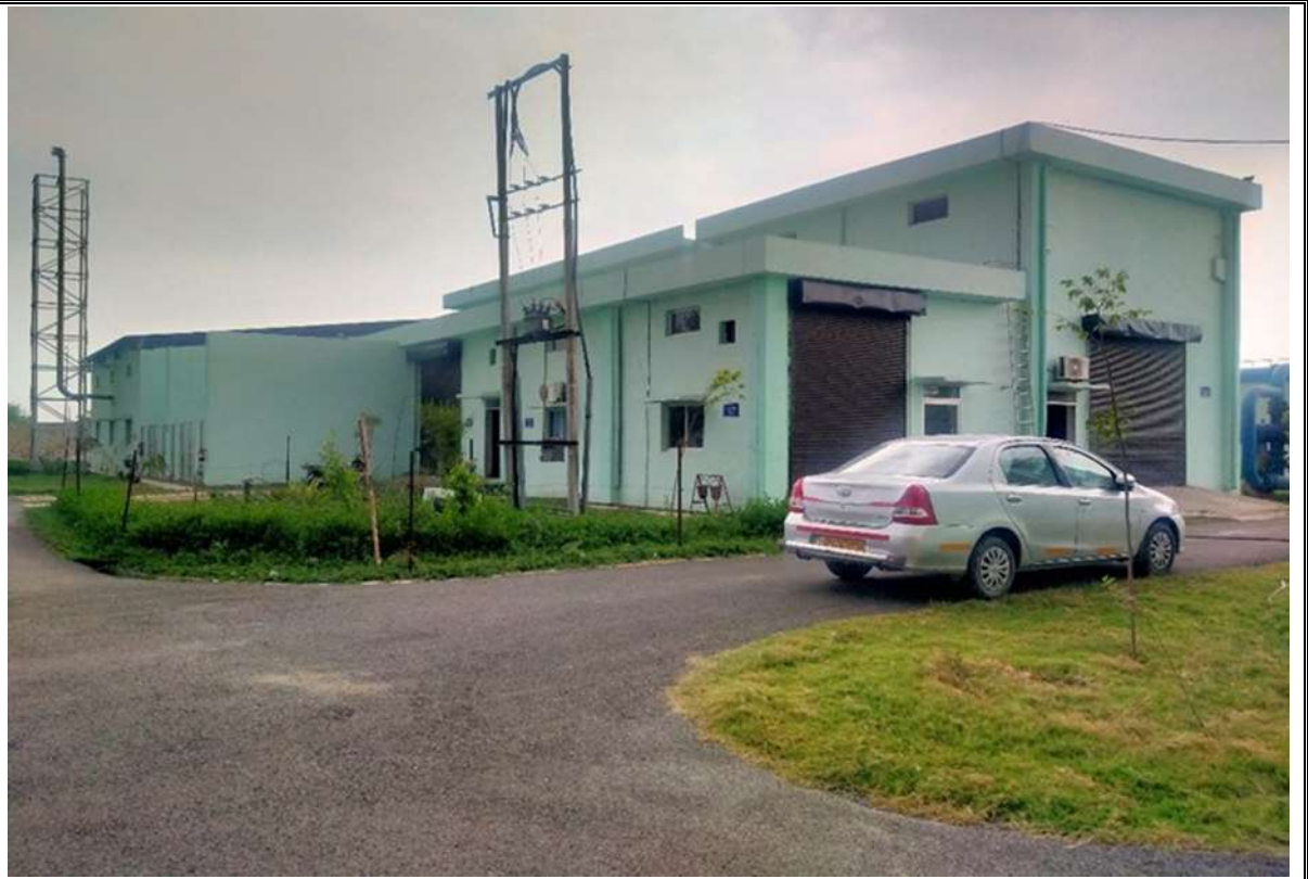
Air blower, HT, PMCC room & DG Shed area
