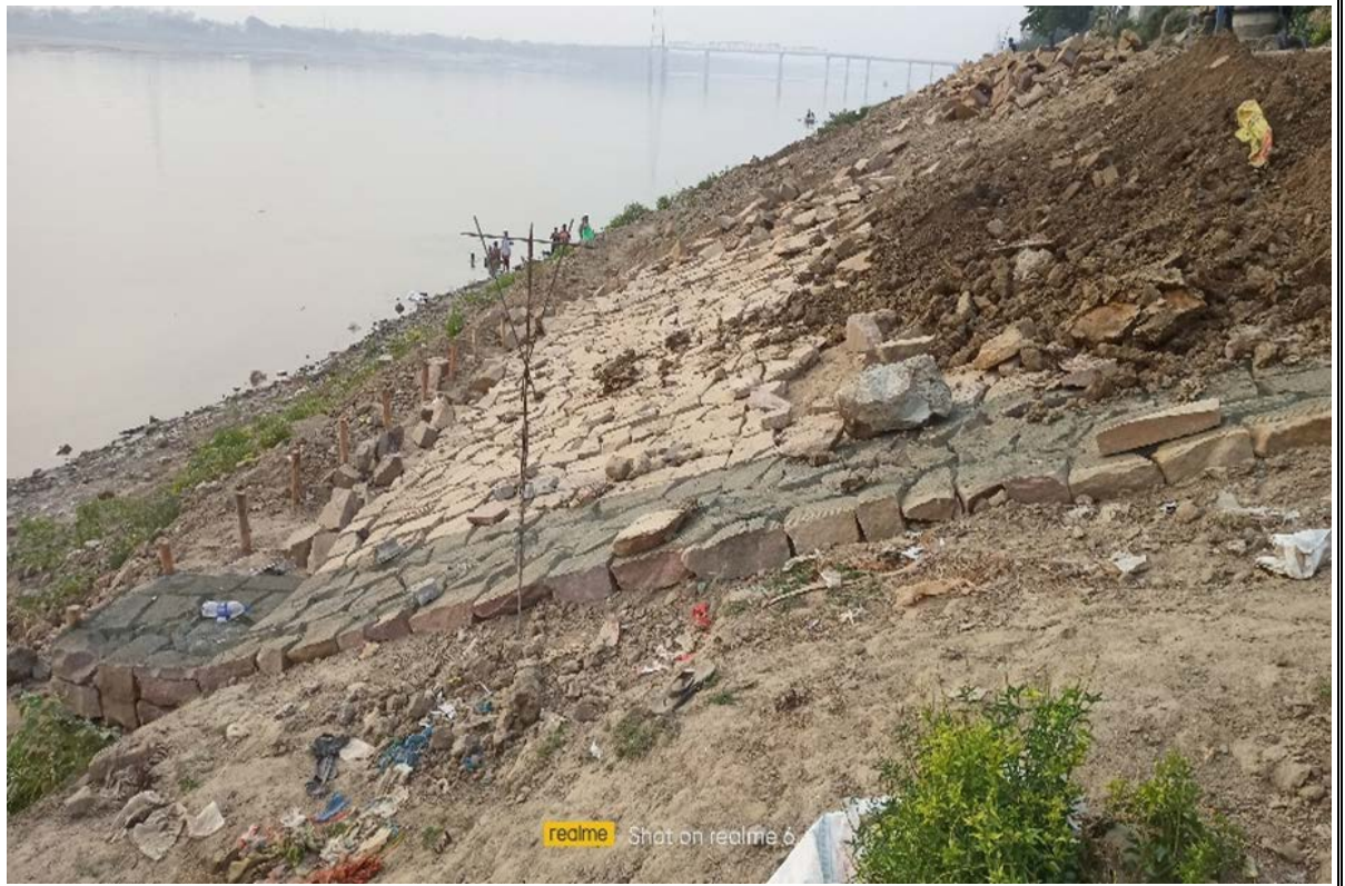
Stone Pitching @ Rising Main near MPS
