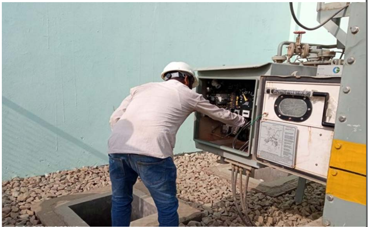
Maintenance work at Transformer, STP
