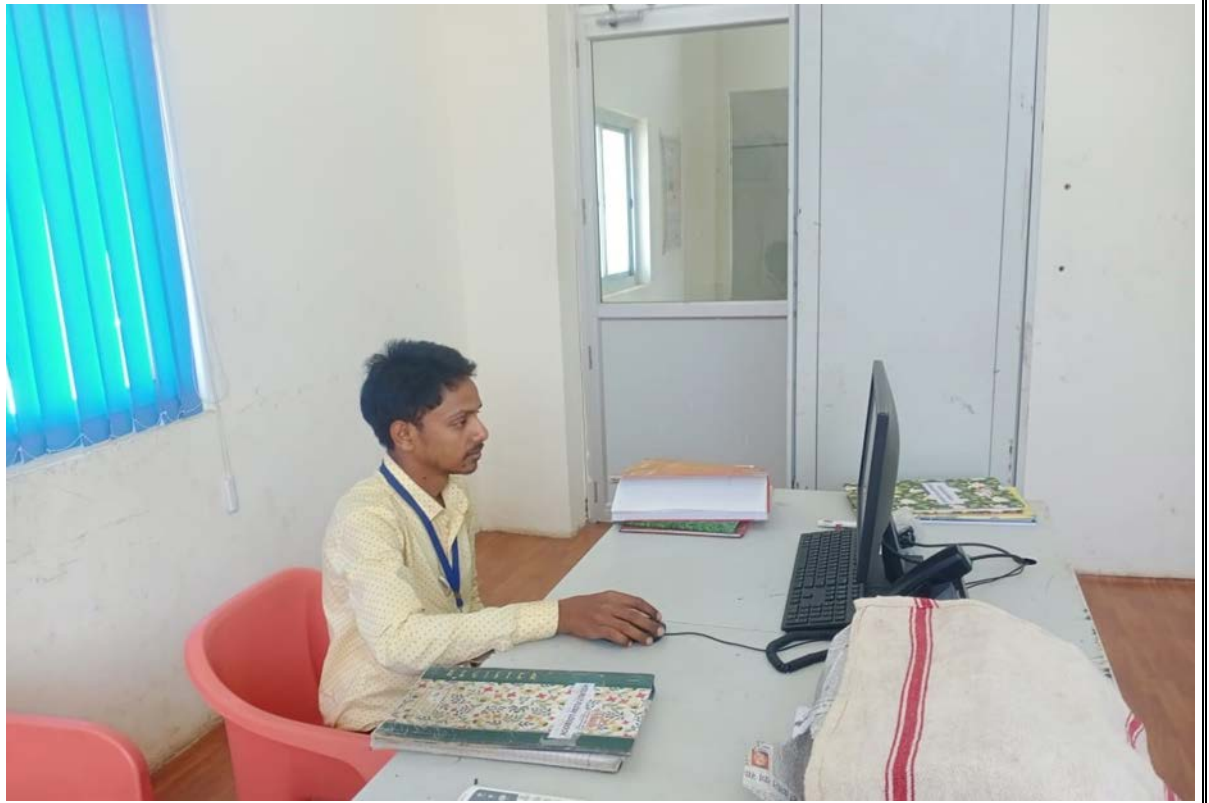
PLC & SCADA Room @ MPS
