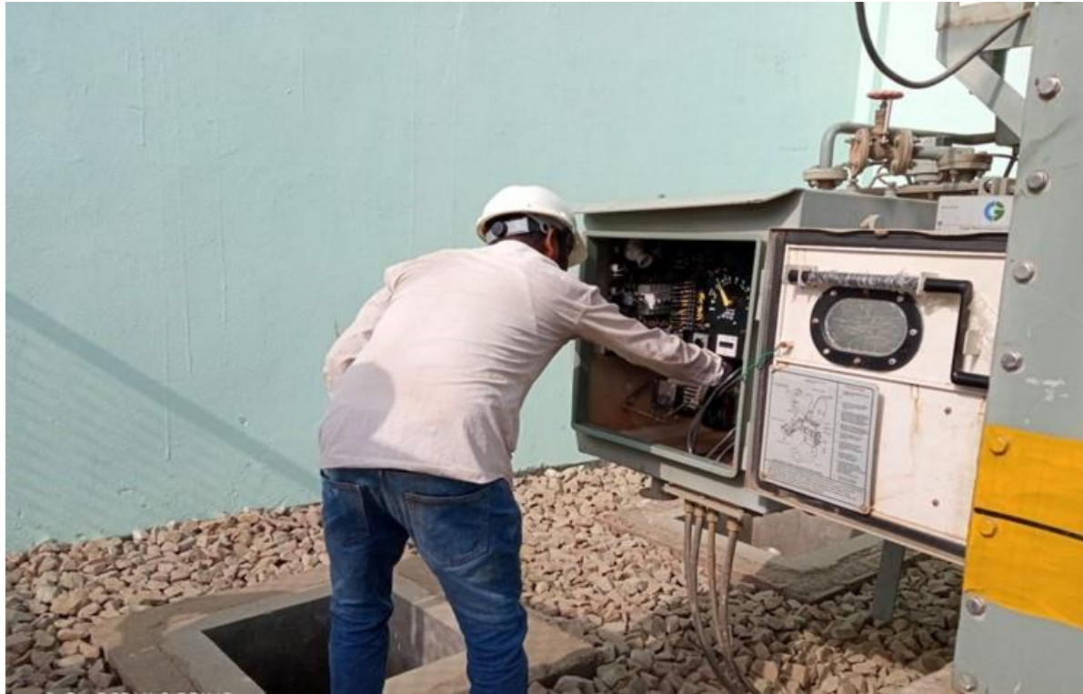
Maintenance work at Transformer, STP
