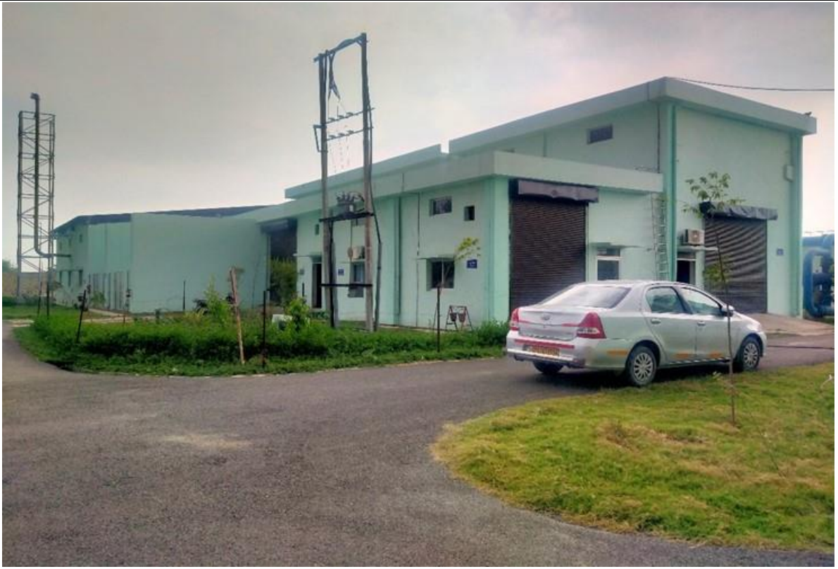
Airblower, HT, PMCC room & DG Shed area
