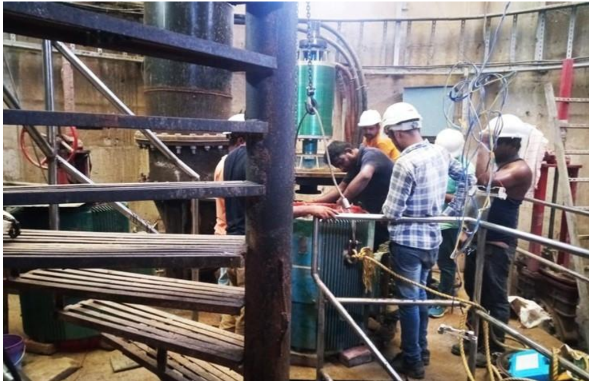
Pumps Repair and Maintenance work @ Dry Well, MPS
