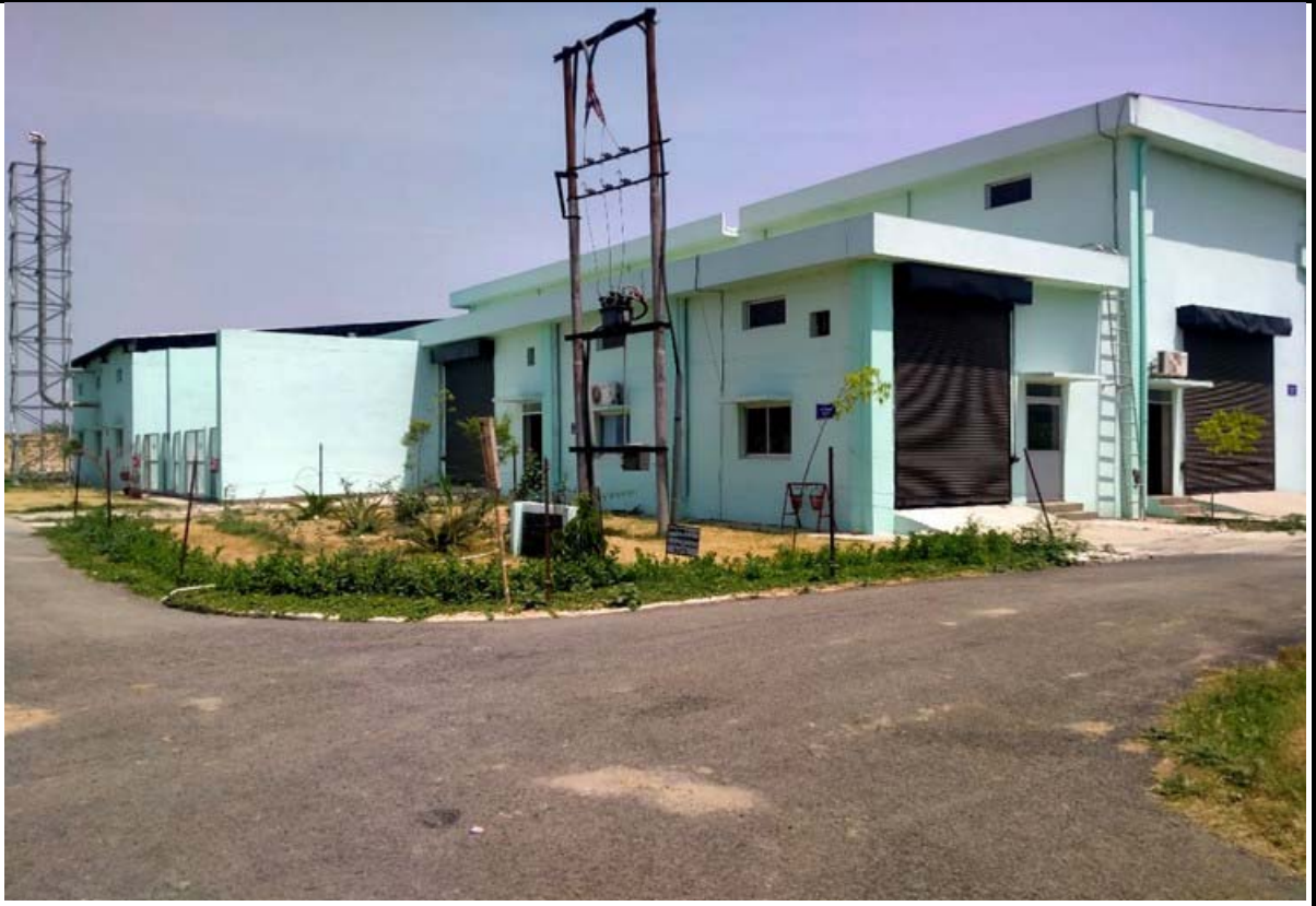
Air blower, HT, PMCC room & DG Shed area
