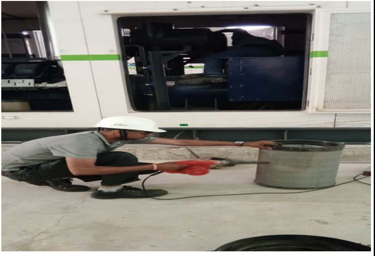
Maintenance work @ DG Set, STP
