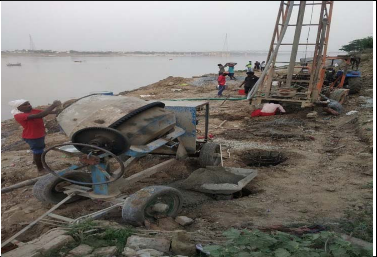
Strengthening work of Rising Main near Ganga Basin
