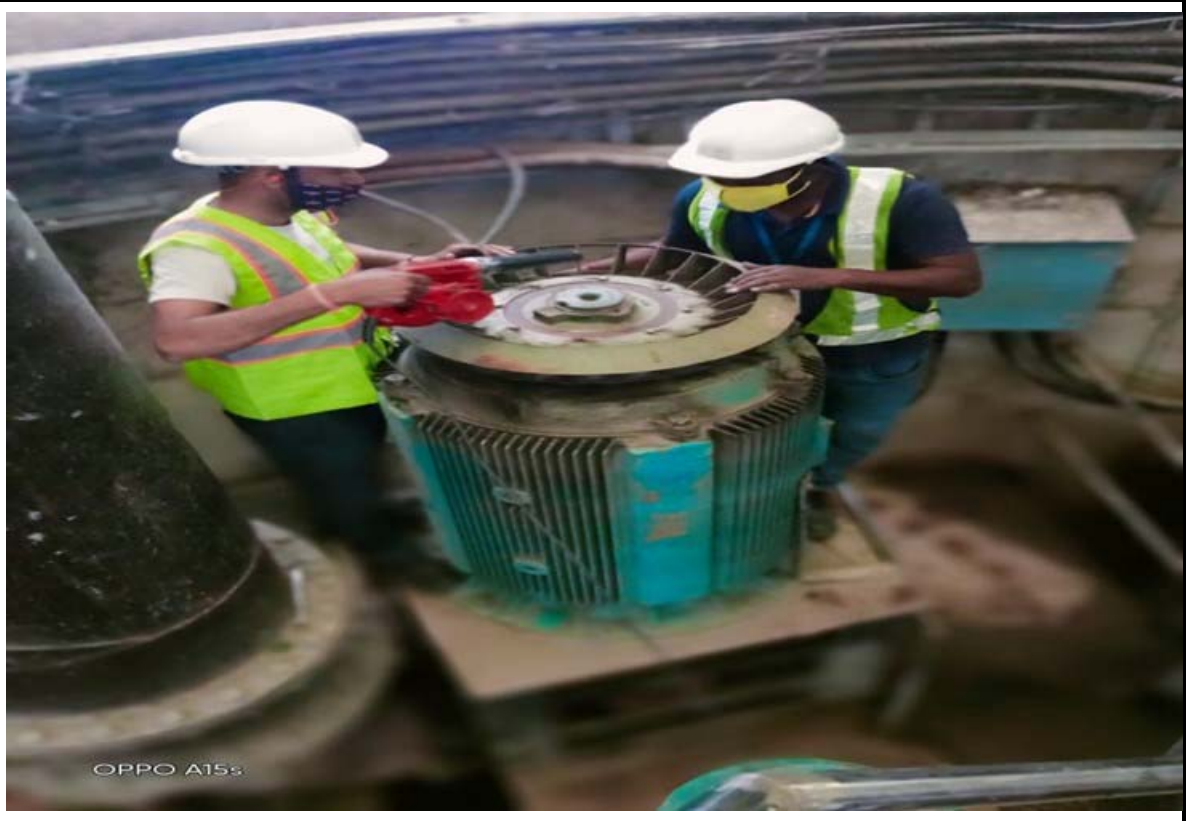
Maintenance work at Pumps
