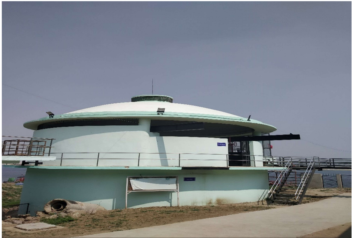
MPS Wet Well and Dry Well
