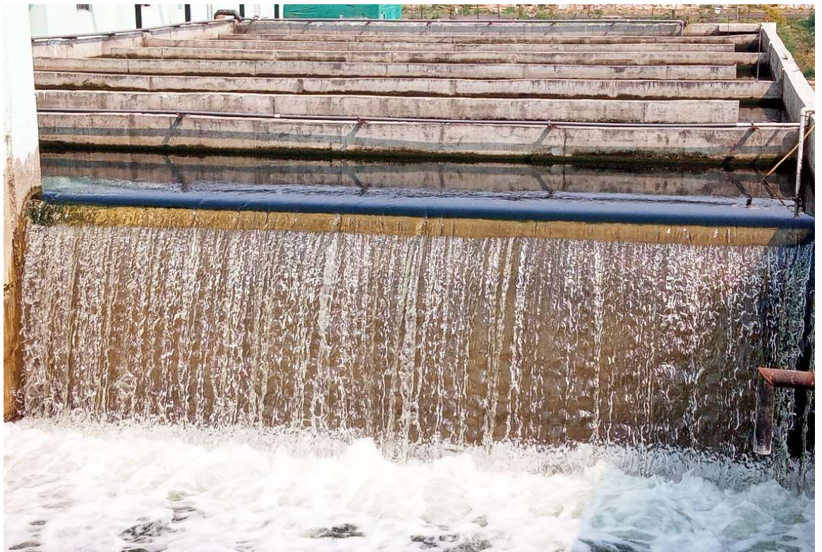
Quality of Treated Effluent at Treated Water Collection Tank ,STP
