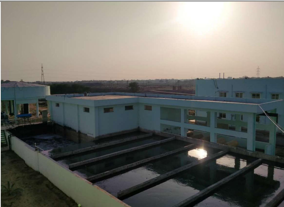
CCT & Tonner Room
