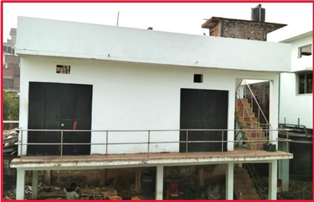
Repair and Rehabilitation of Existing Building
