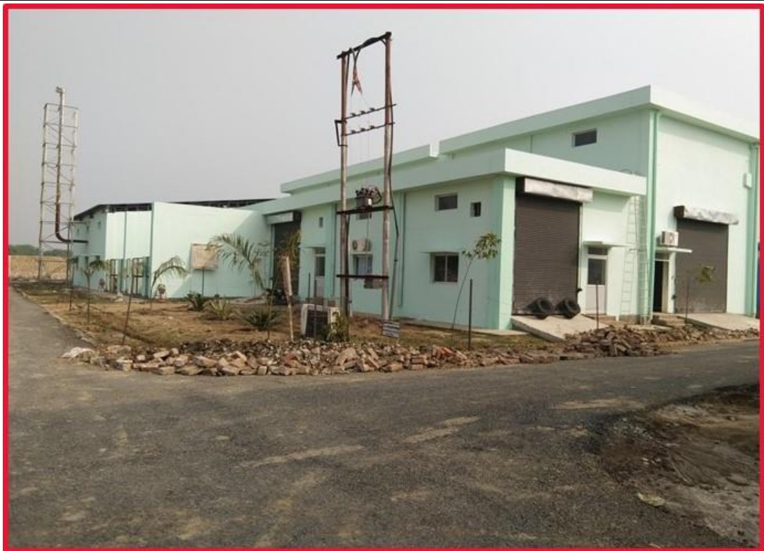
Airblower, HT room, MCC, PMCC & DG Shed
