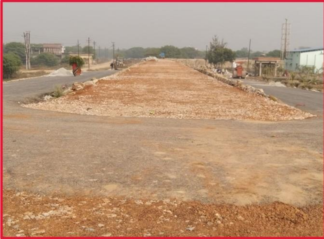
Approach Road and Path Way over the Bund Wall
