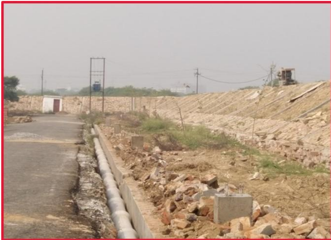
Lighting Pole foundations @ STP
