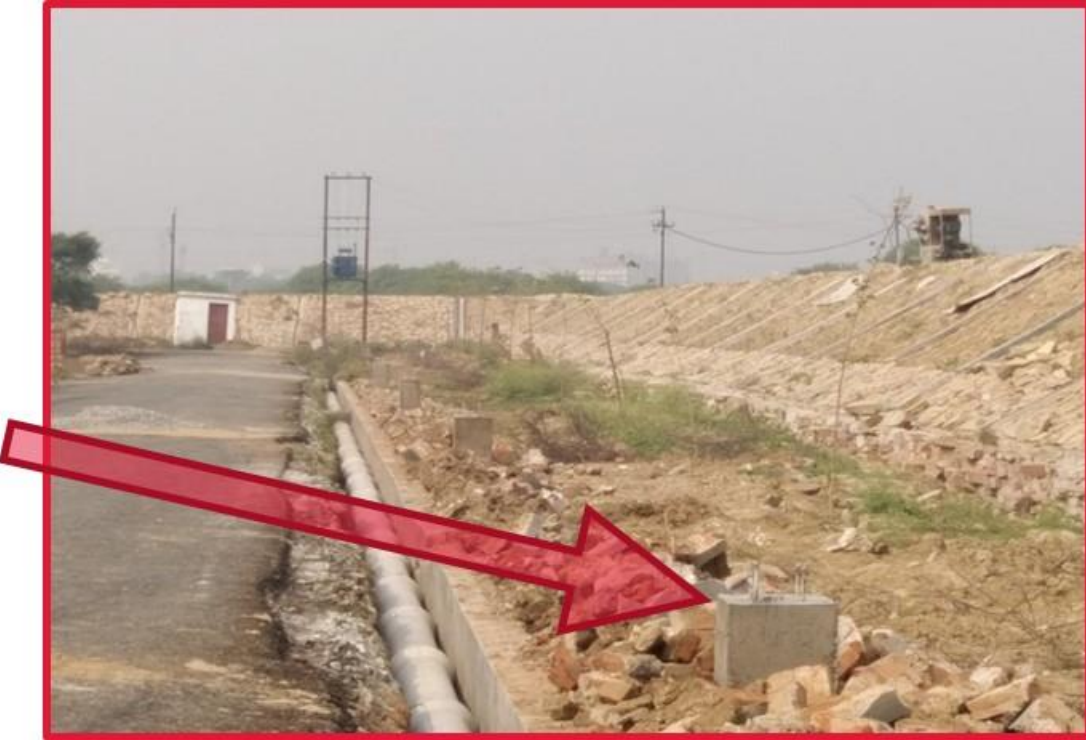
Lighting Pole foundations @ STP
