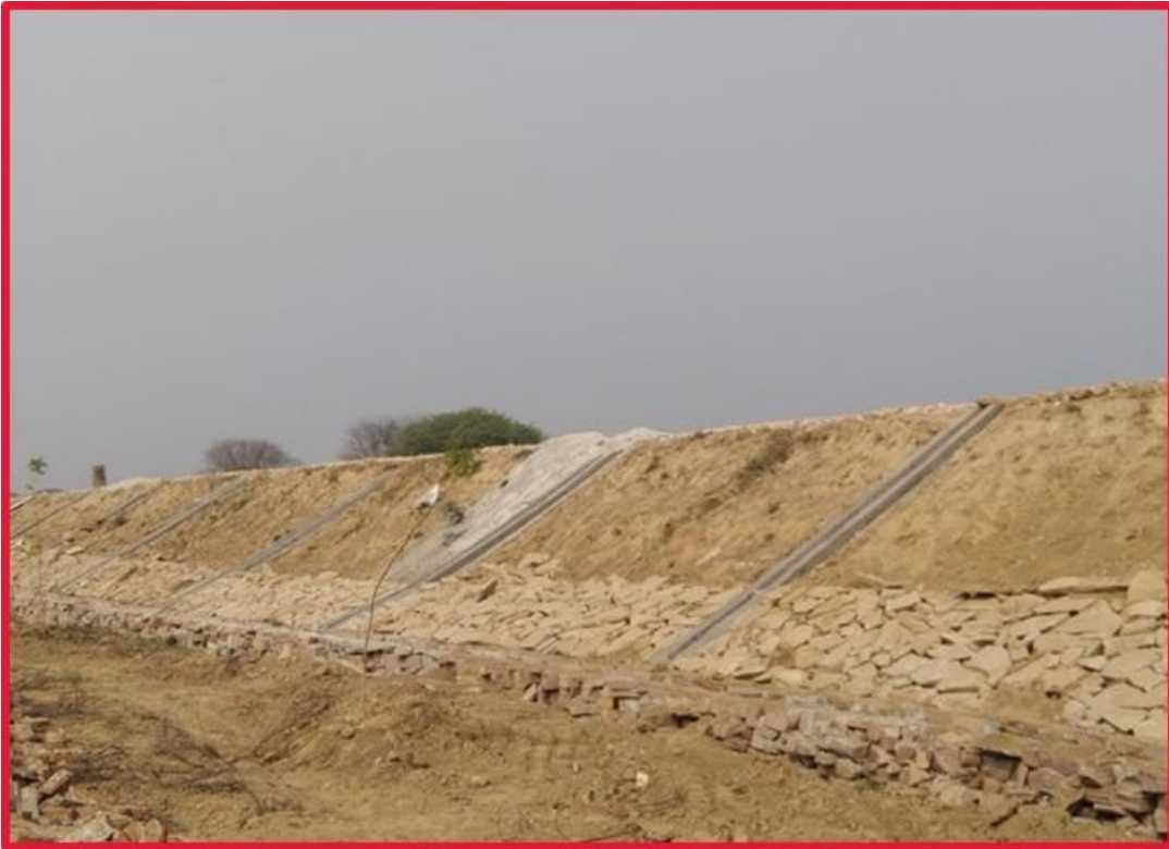
Stone Pitching With Drain @ Bundwall
