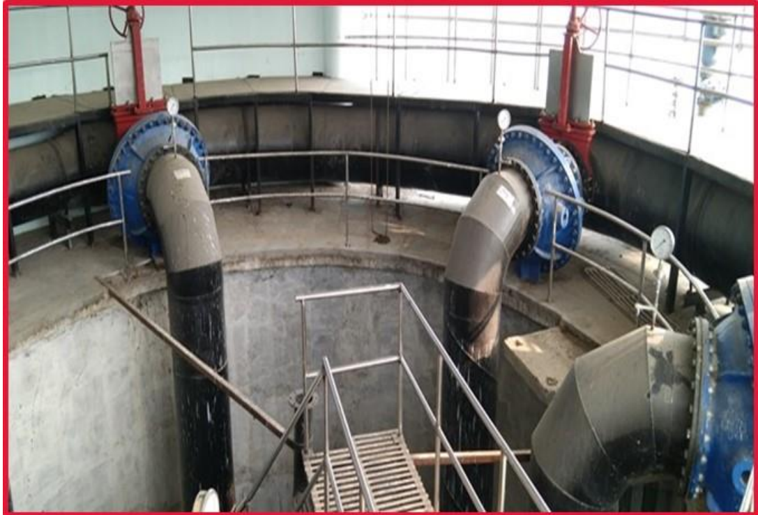
Common Header Line , MPS
