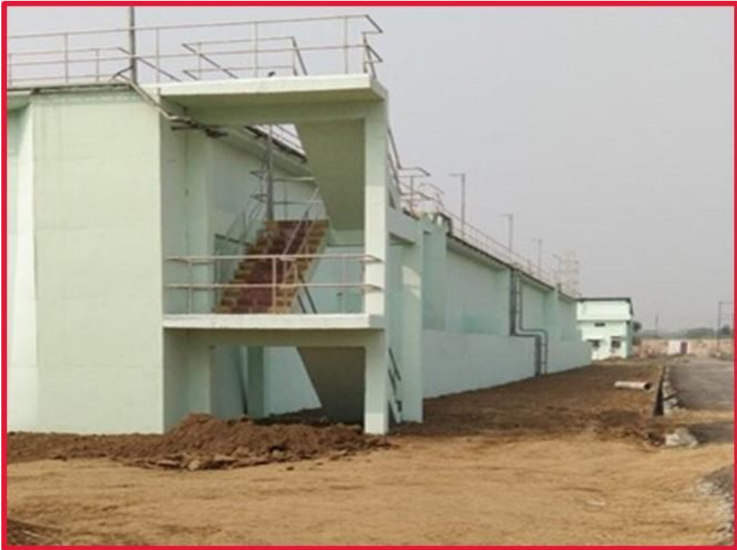
Site Grading @ STP
