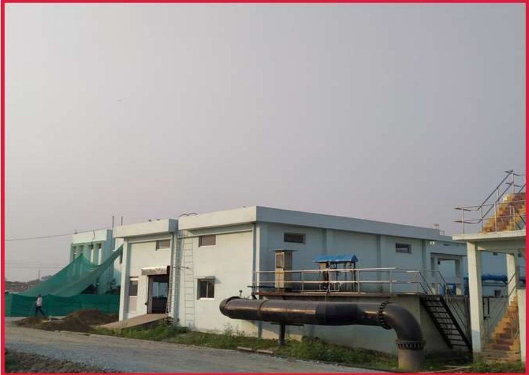
Treated Water Pump House
