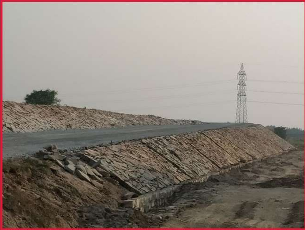
Stone Pitching @ Outer Side Bund Wall
