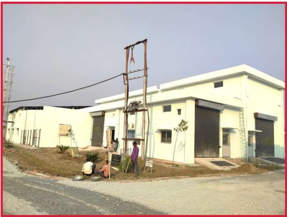
Airblower, HT room, MCC, PMCC & DG Shed
