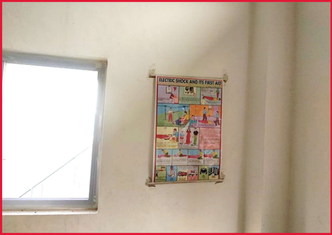
Safety Signage Board @ Panel Room, MPS
