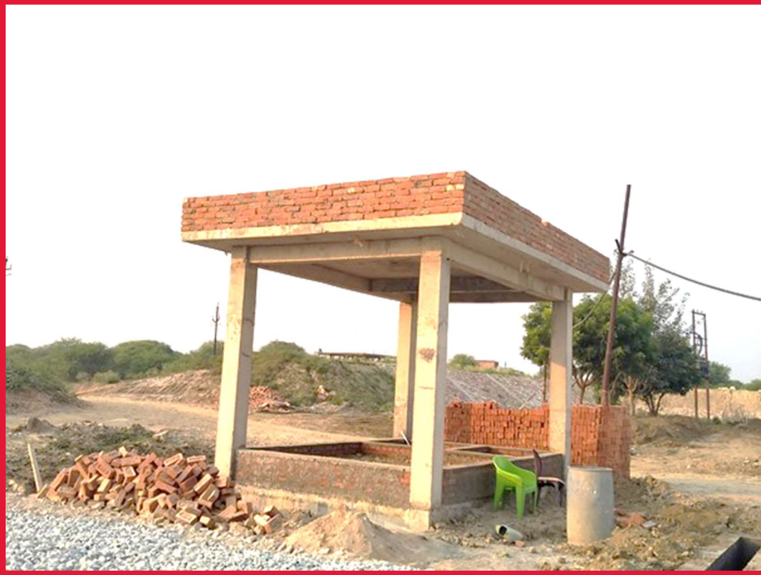
Security Building, STP
