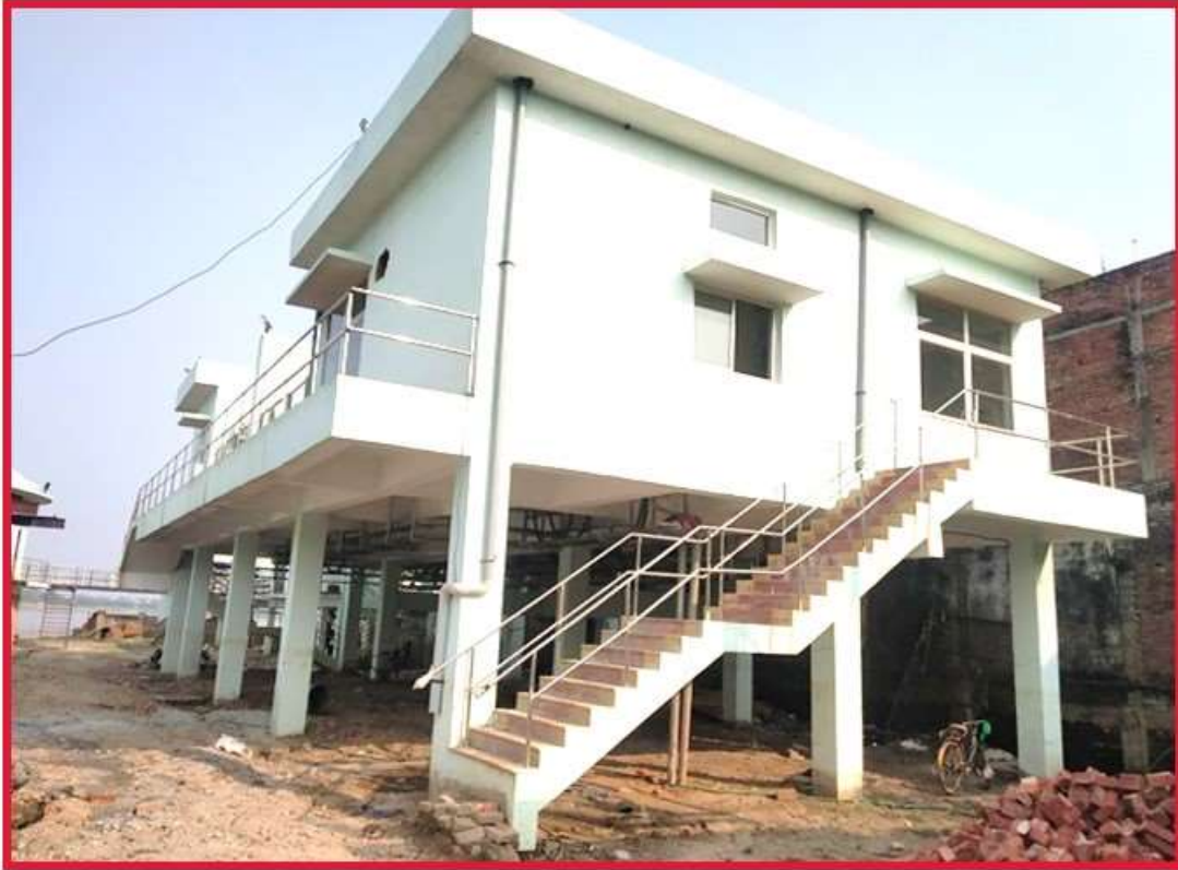
Electrical control building at MPS
