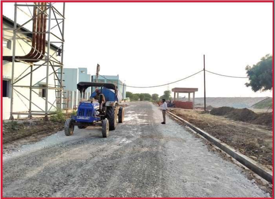
STP Area Internal Road Work
