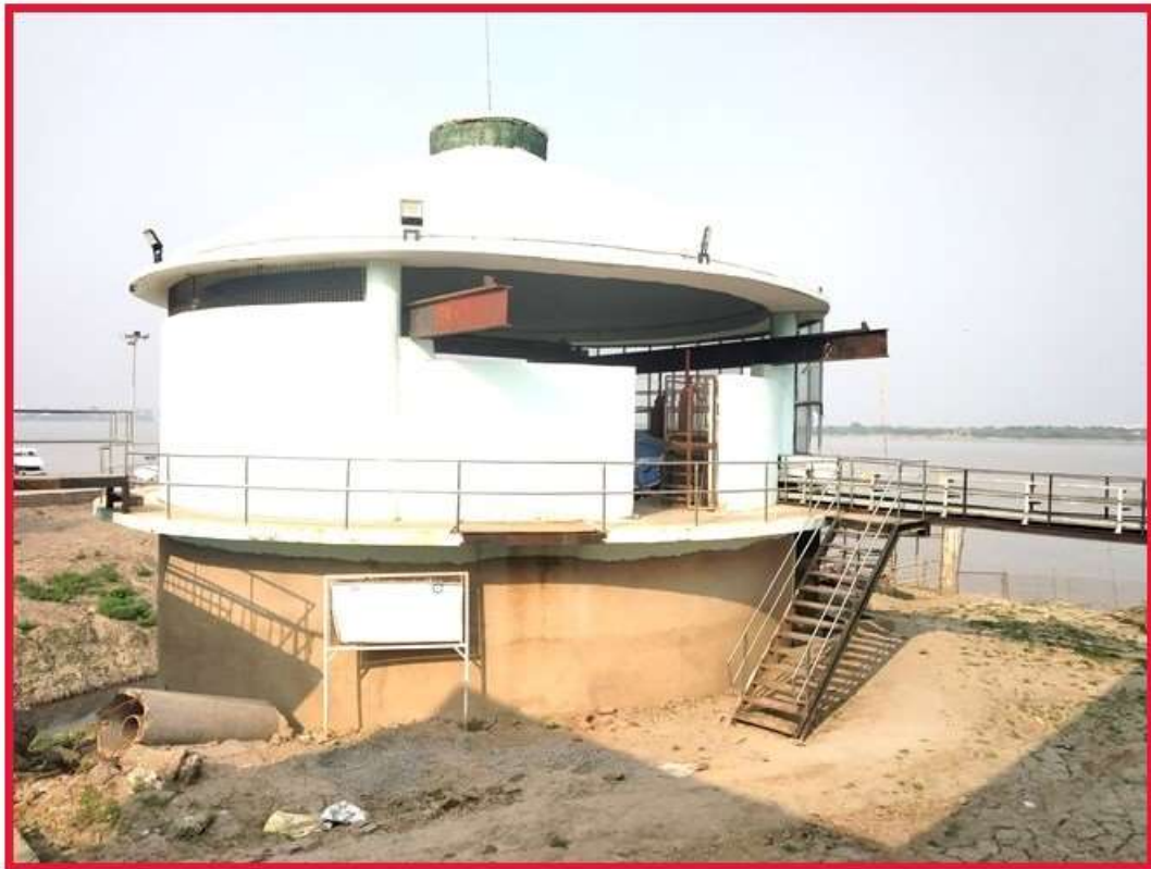
MPS Wet Well and Dry Well,
