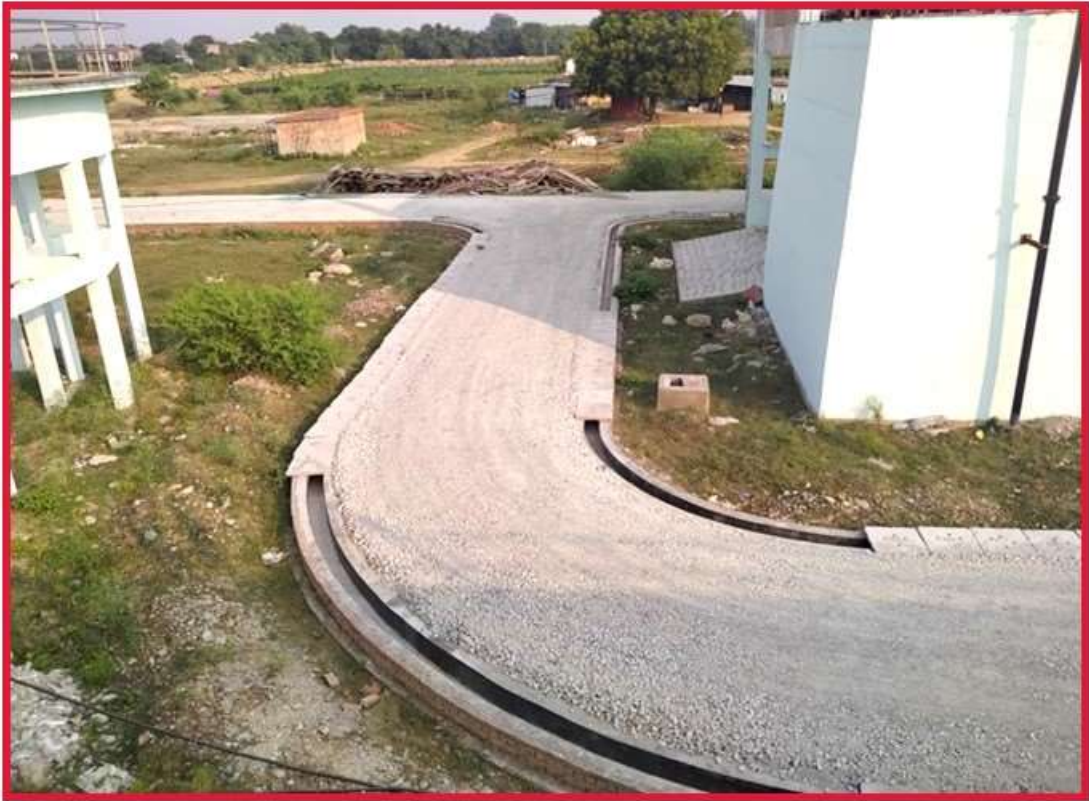
Top layer of WBM laid @ Road Work
