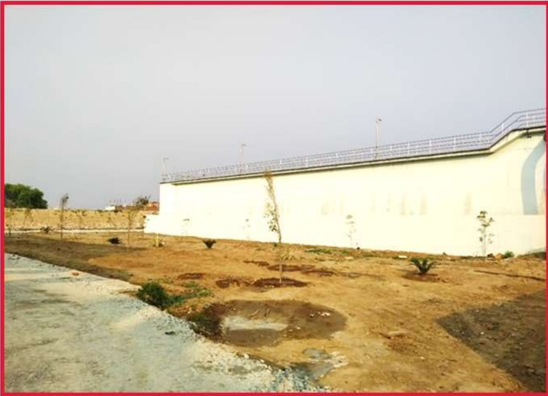
Landscaping work @ STP
