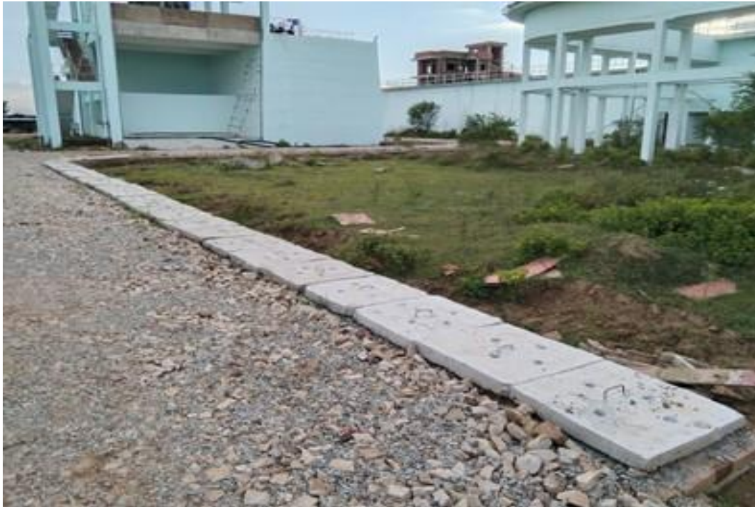
Drain with Cover slab
