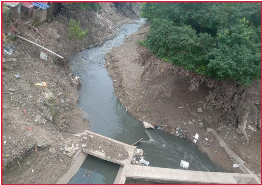
Weir Across Assi Nala
