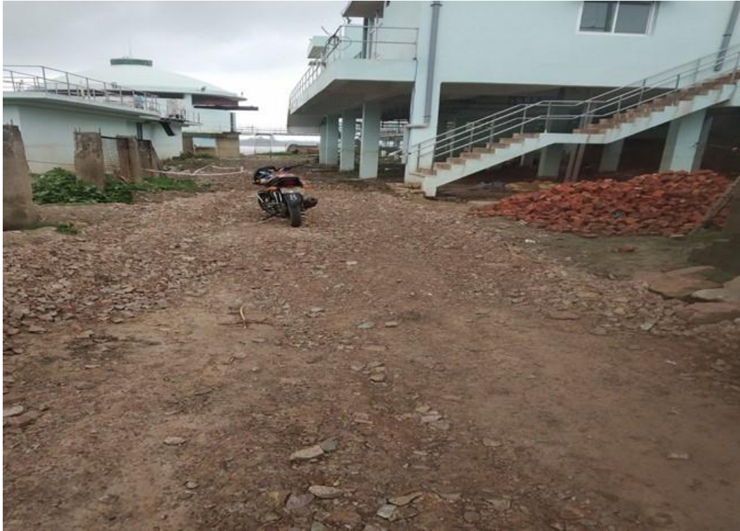
WBM laying at MPS
