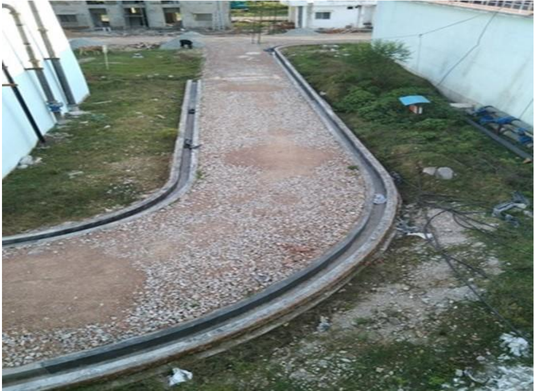
Road Work @ STP
