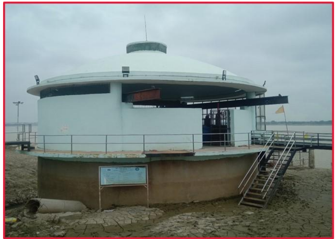
MPS Wet Well and Dry Well,
