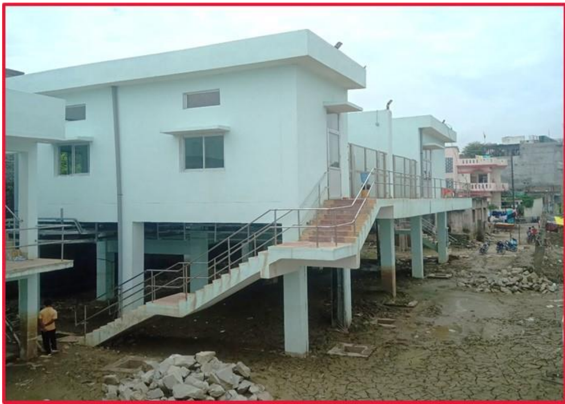
Electrical control building at MPS
