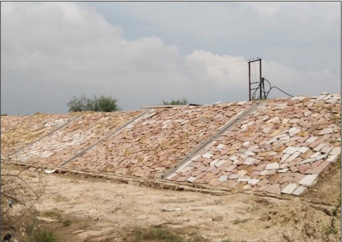
Stone Pitching @ West Side Bund Wall
