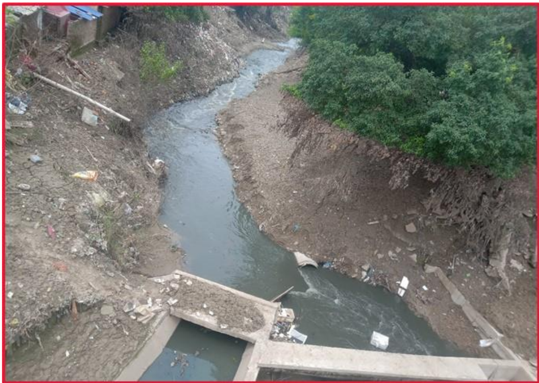
Weir Across Assi Nala
