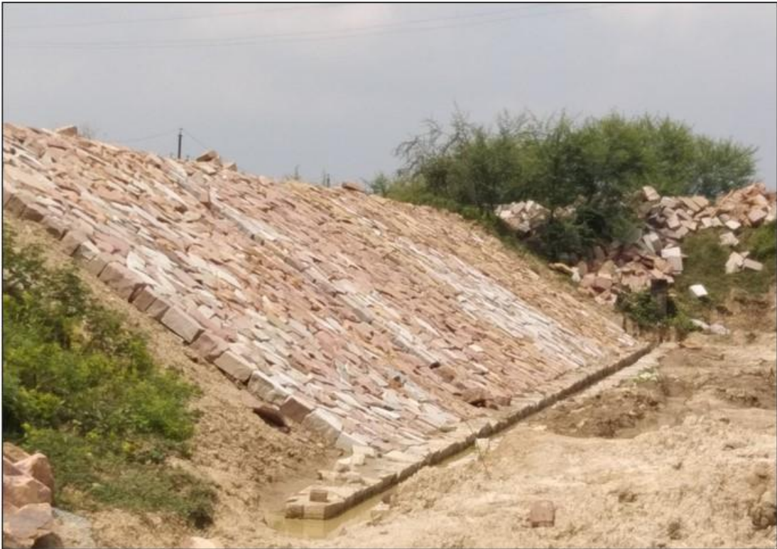
Inner Stone Pitching @ West Side Bund Wall
