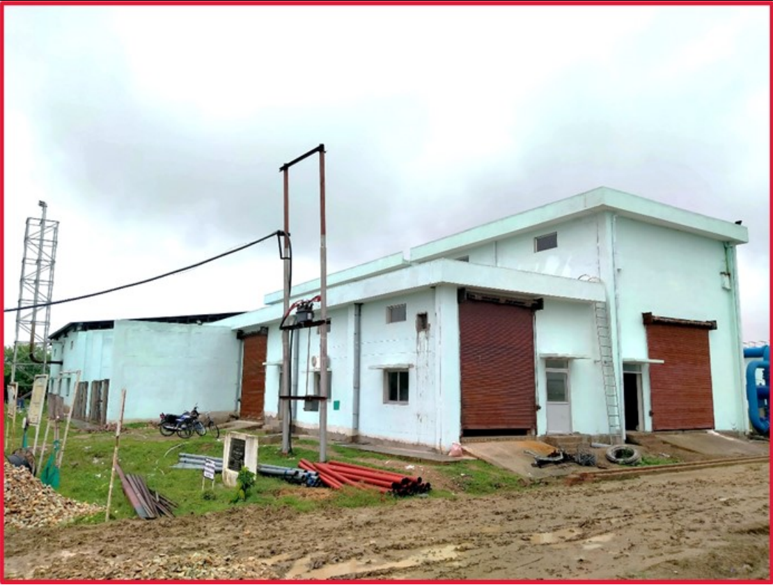
Airblower, HT room, MCC, PMCC & DG Shed
