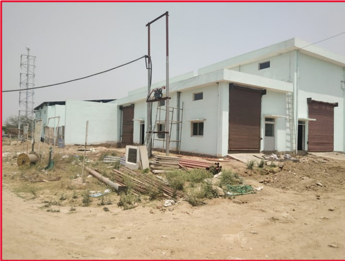
Airblower, HT room, MCC, PMCC & DG Shed
