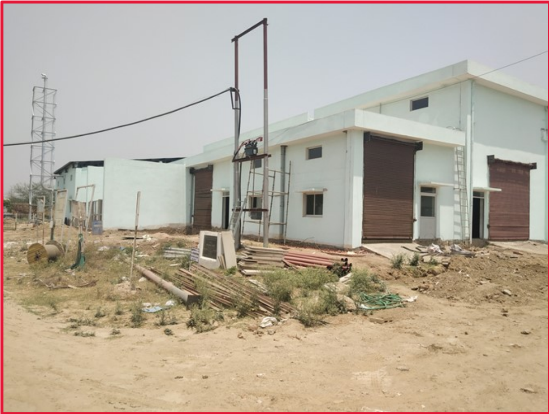
Airblower, HT room, MCC, PMCC & DG Shed
