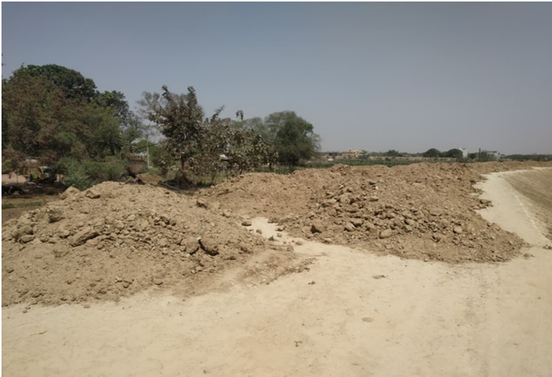
Earth Filling @ East Side Bund Wall
