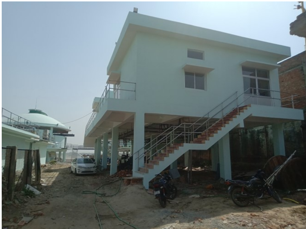
Electrical control building
