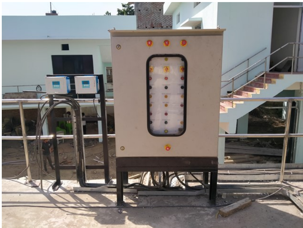
Erection of LDT Controller & Panel for Coarse Screen
