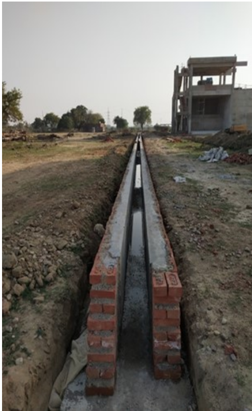
Drain & Road work
