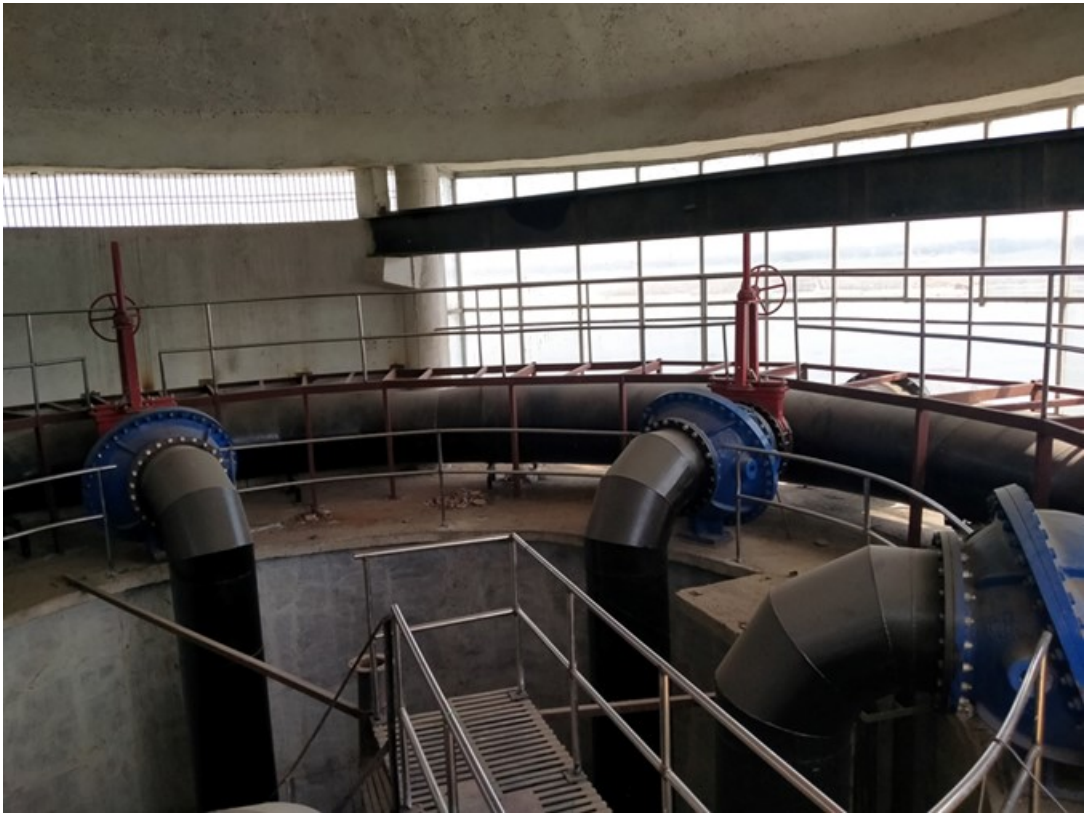
Railing work at Common Header Line, Dry well @ MPS
