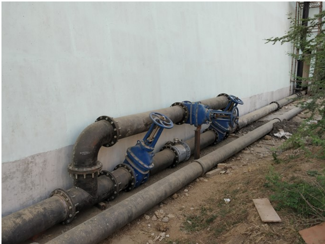
Flowmeter erection at STP Site
