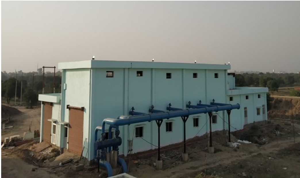
Airblower, HT room, MCC, PMCC & DG Shed
