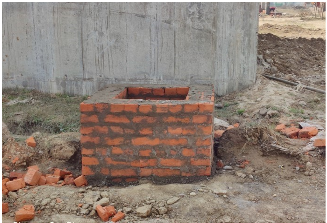
Earthing Pit Chamber Brick work @ STP
