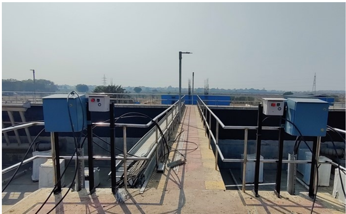
Fixing of LPBS & Power JB @ STP
