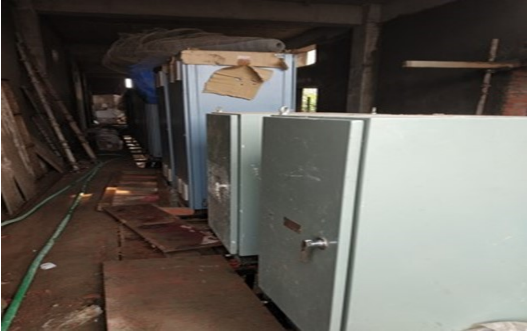
Panel erection at Electrical control Room, MPS
