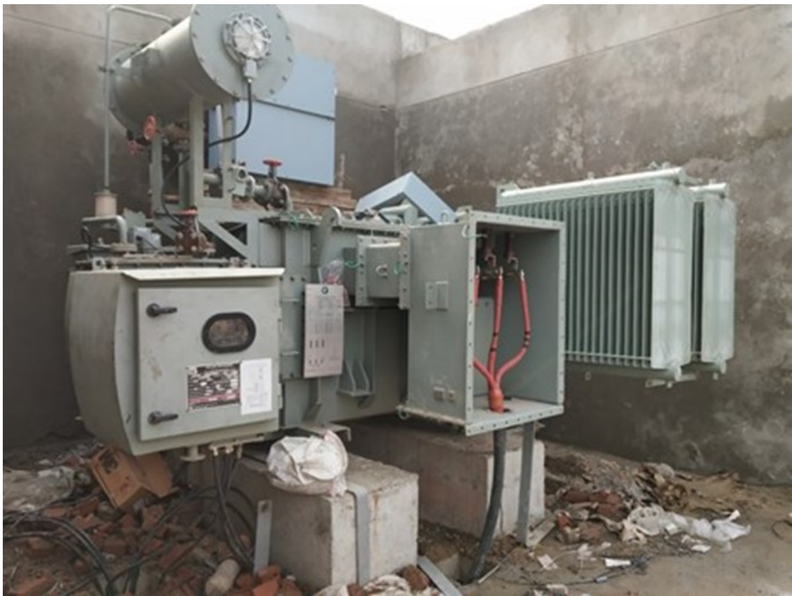
Transformer erection at Electrical Control Room, MPS
