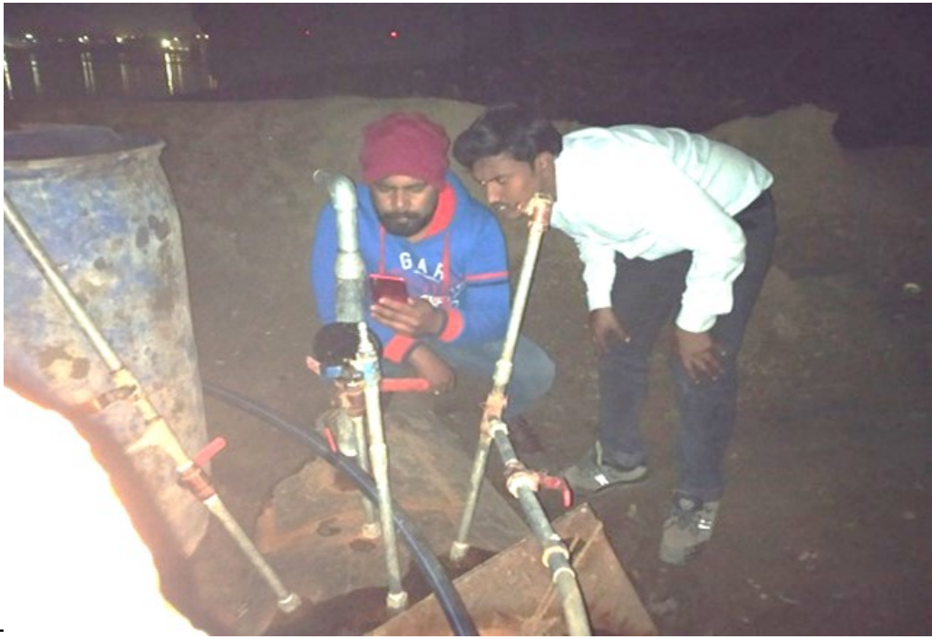
Rising main - Measuring of Water Consumption in Hydrotest
