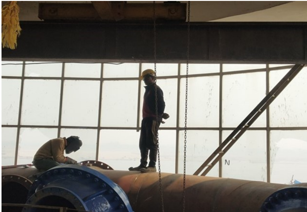
Pipe Welding Work on Common Header Pipe @ Dry Well, MPS
