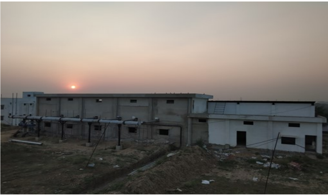
Airblower, HT room, MCC, PMCC & DG Shed
