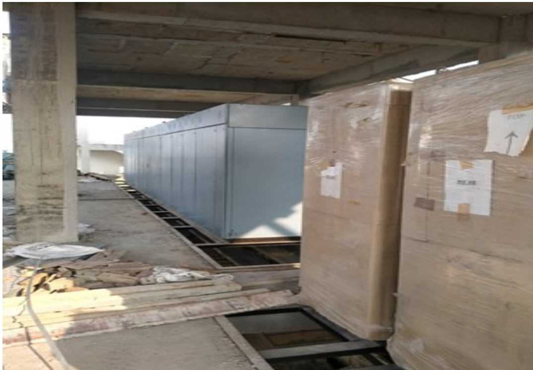
Panel erection – Electrical control room
