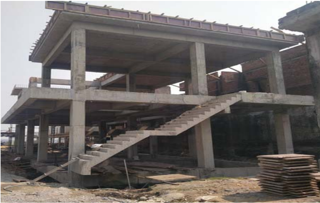
Electrical control building
