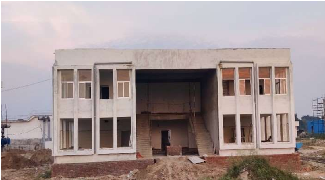
Admin building – Front view
