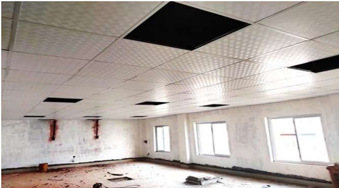
Admin building – False ceiling
