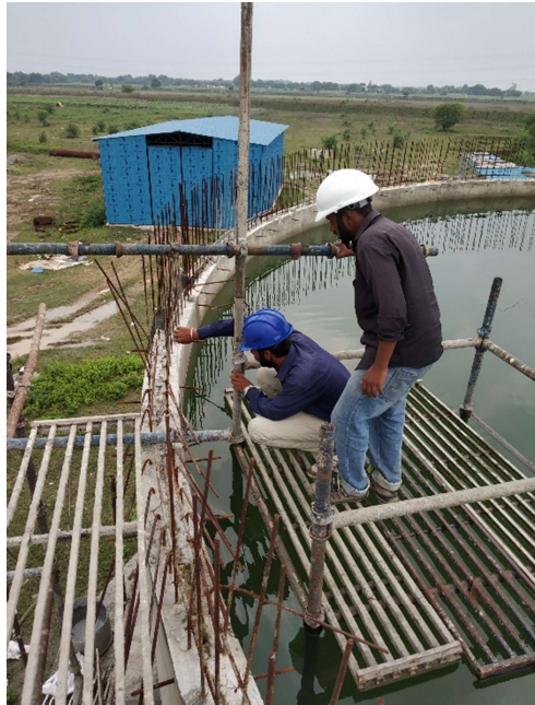
Hydro testing and Thrust Block at OHT
