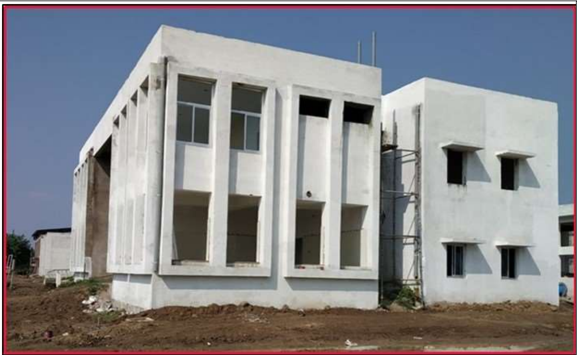
Admin building – Side view
