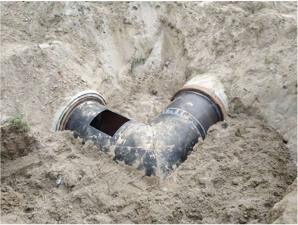
Treated Effluent pipe line – Gap closing work
