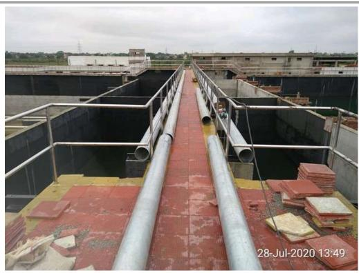
SBR basin - Surplus activated sludge pipe laying
