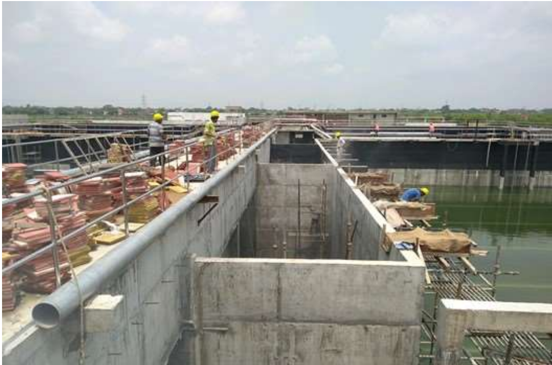
SBR basin 1 & 2 - Air header pipe laying 1
