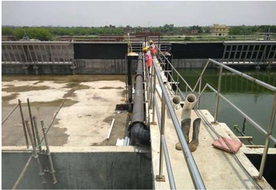
SBR basin 2 - Surplus activated sludge pipe laying
