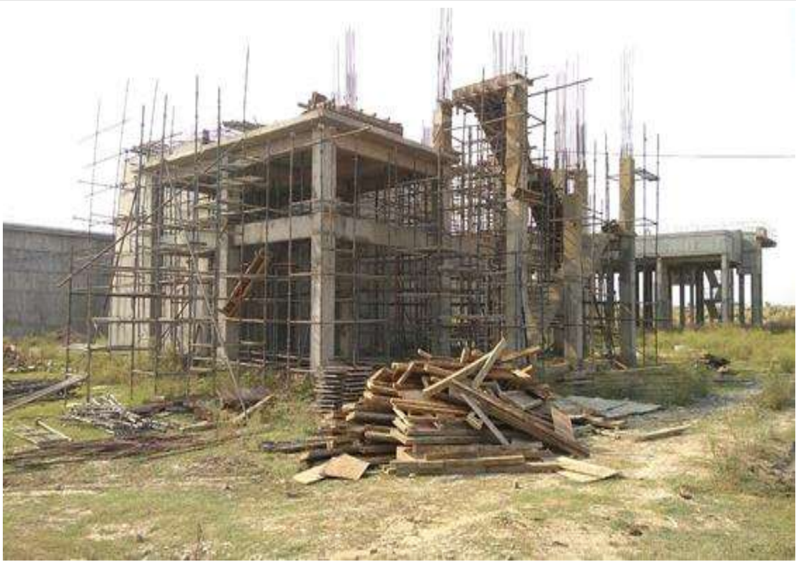
Sludge treatment building
