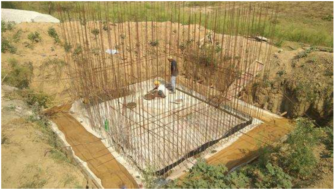
Final outfall chamber
