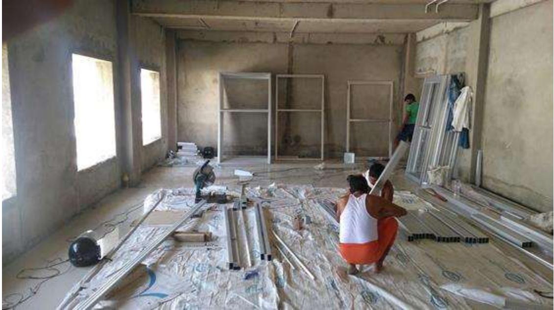
Admin building – Doors & windows fabrication
