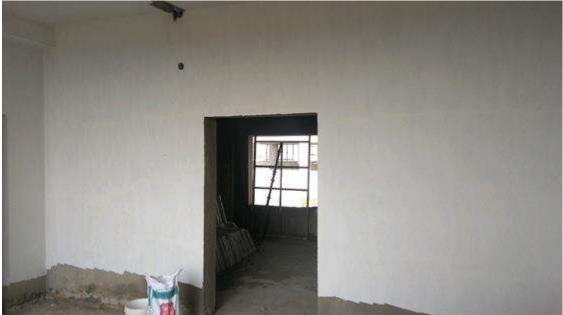
Admin building – Painting
