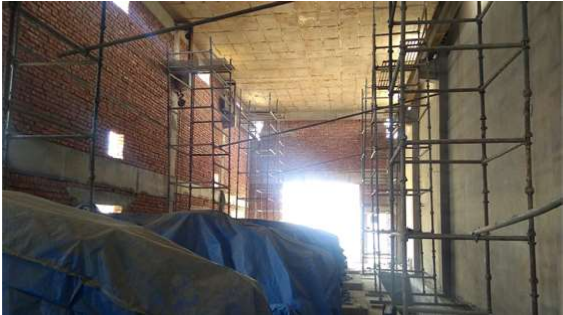
EOT girder erection at air blower building
