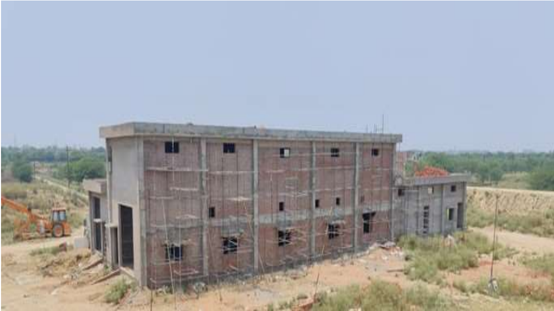
Air Blower & MCC Room Building
