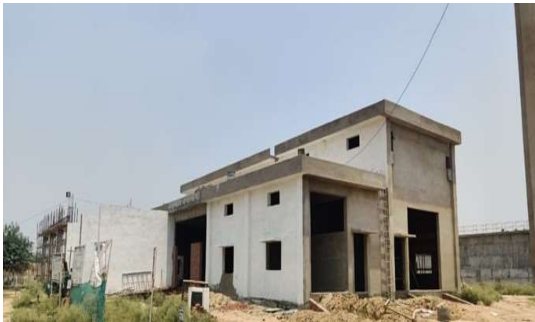
Air Blower & MCC Room Building
