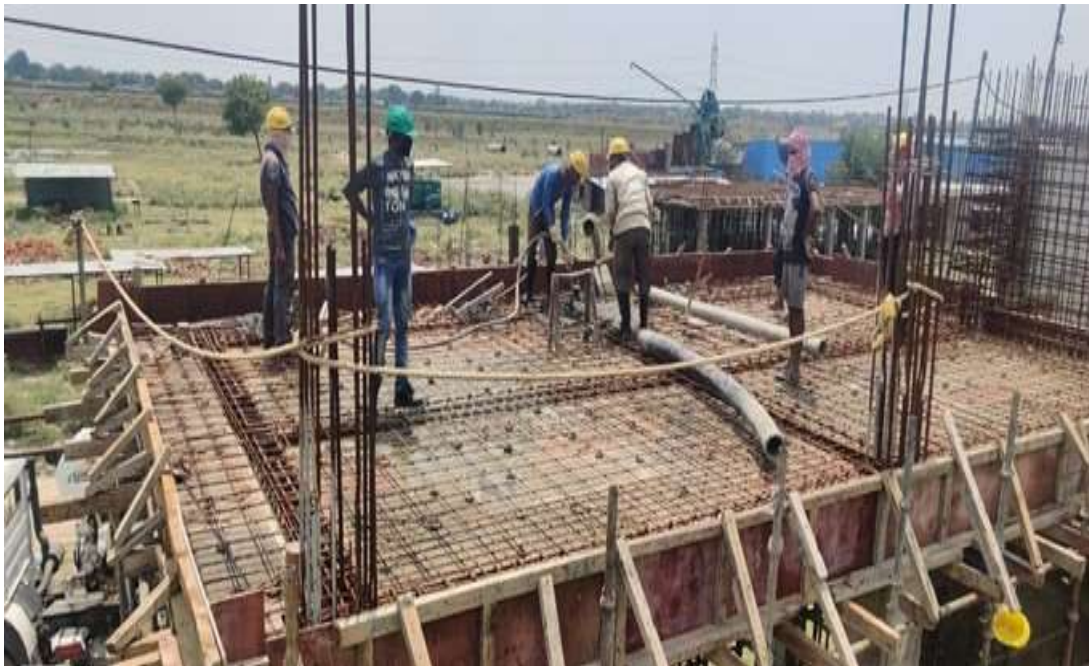
Sludge Treatment Building (02.05.2020)
