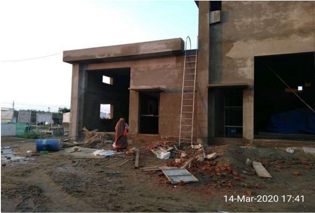
Air Blower Building – Plastering work
