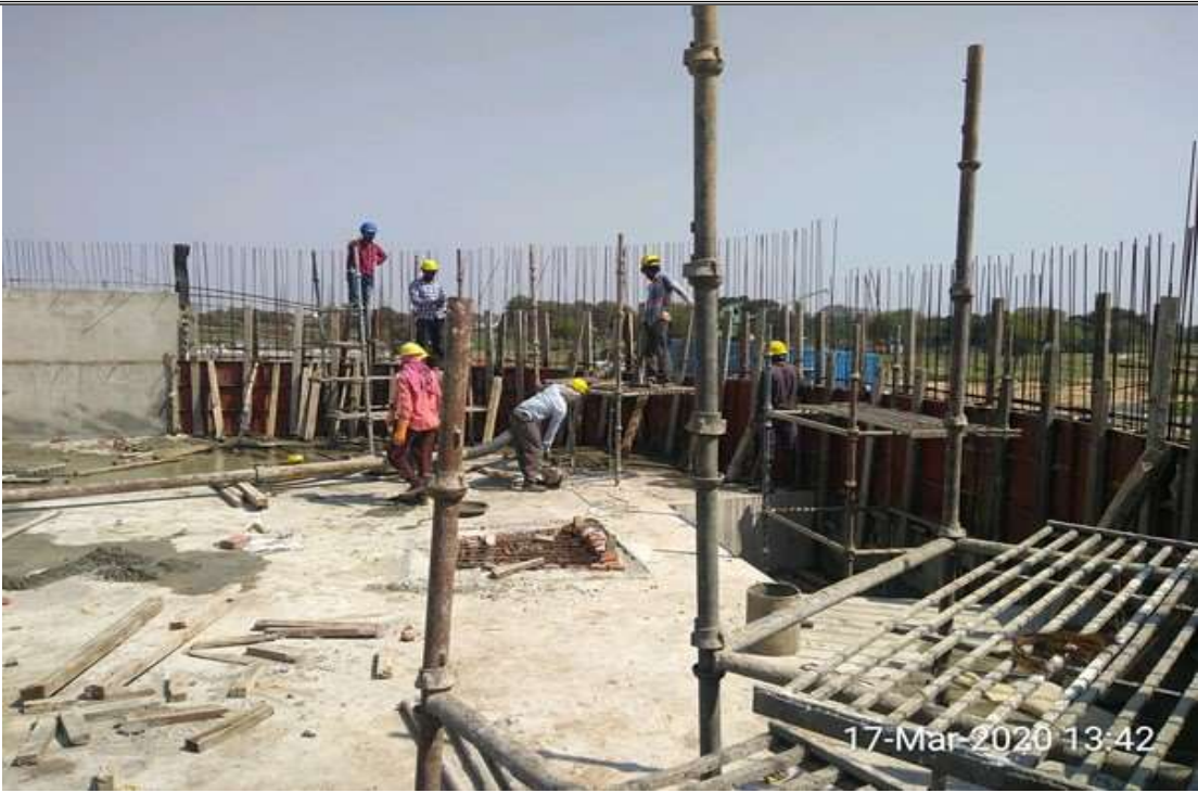
Over Head Tank (OHT)- RCC wall
