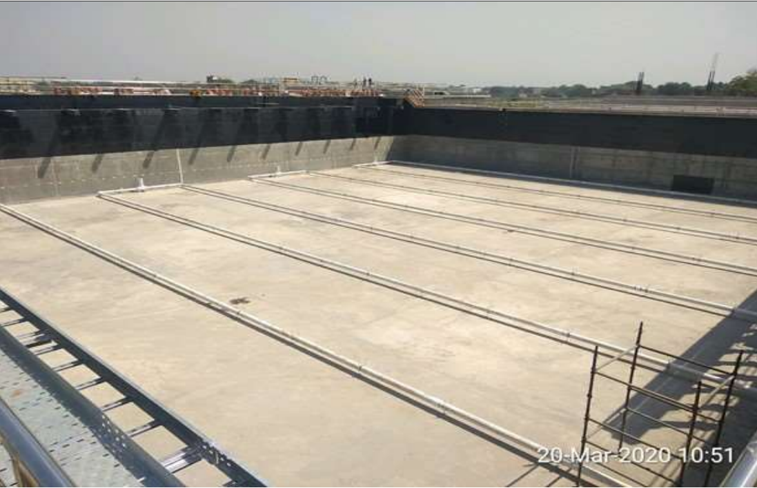
SBR -B4- Cable tray & Piping
