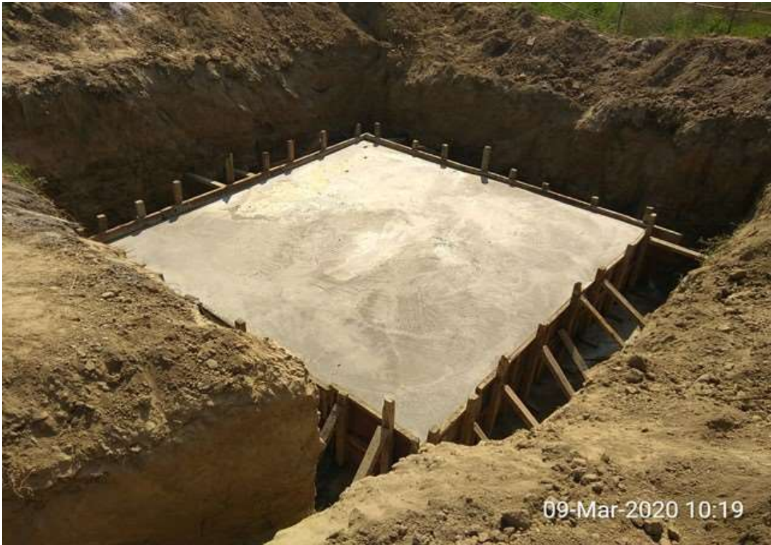
Final outfall chamber - Foundation
