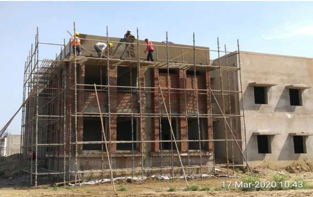
Admin building – External plastering
