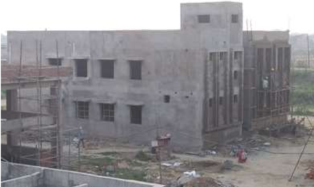
Admin building – External plastering
