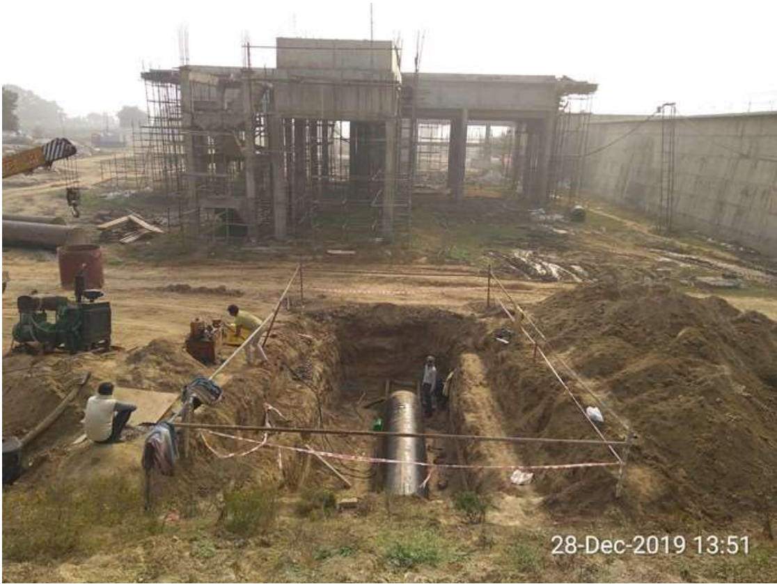
Rising main – STP to Inlet chamber
