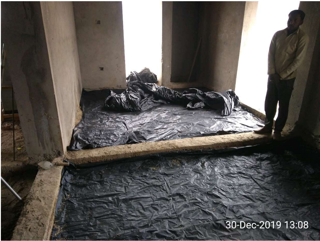
Staff Quarters – Type 4- Flooring PCC
