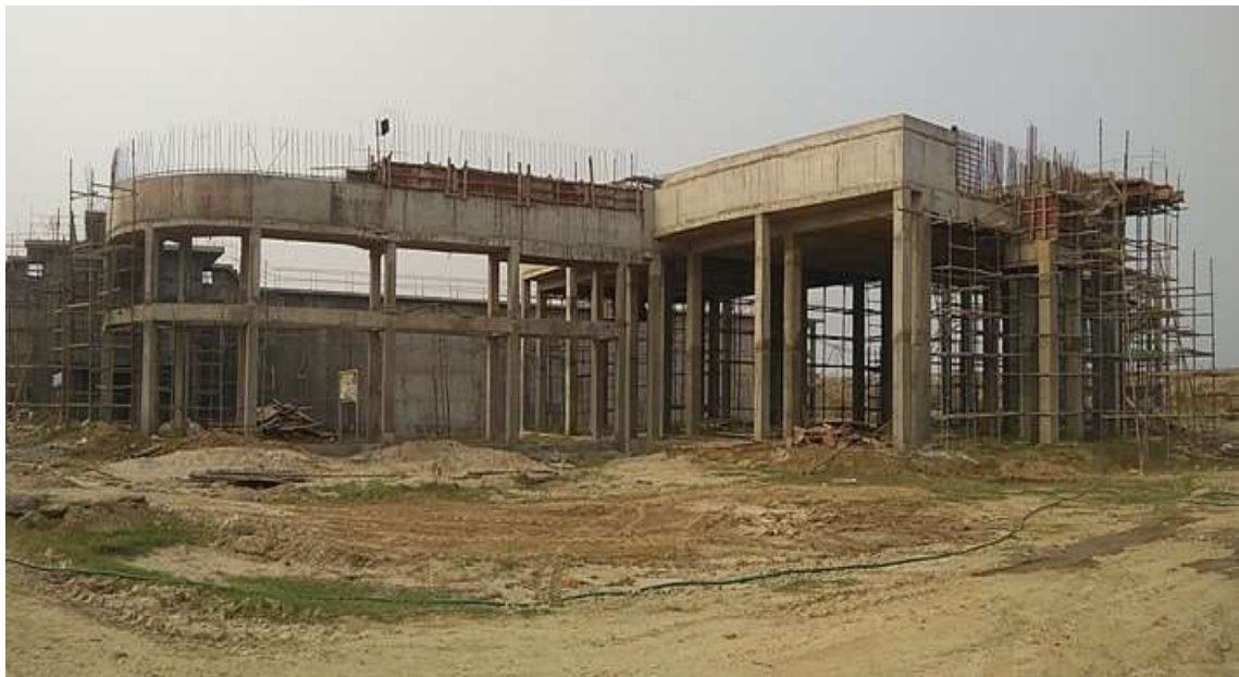
PTU – Parshall Flume
