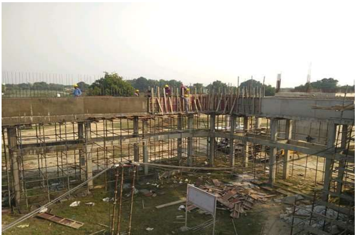
PTU - Parshall Flume
