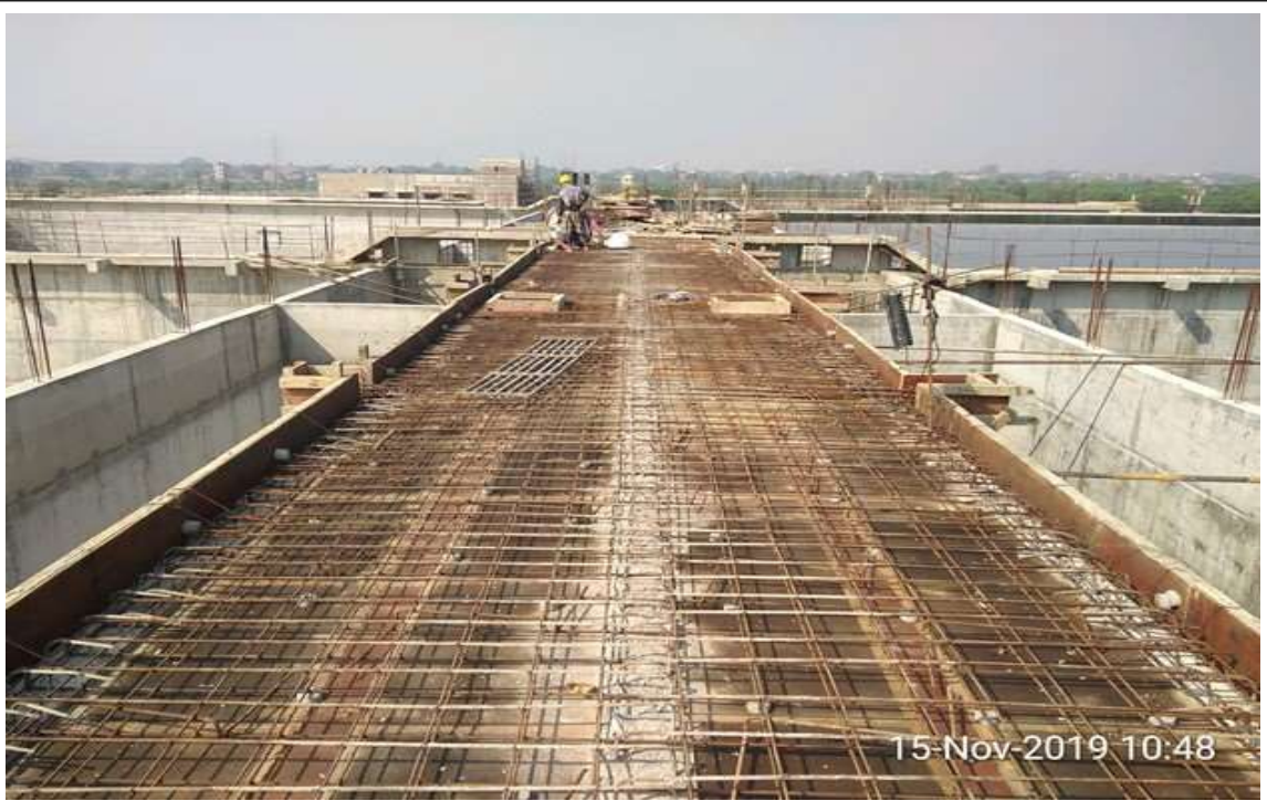
SBR Inlet channel slab
