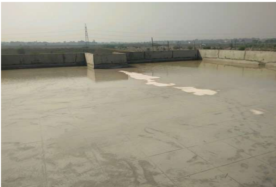
Admin building - After brick coba work
