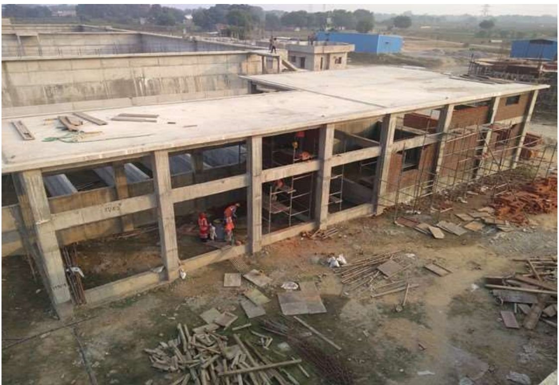
CCT - Treated water pump house
