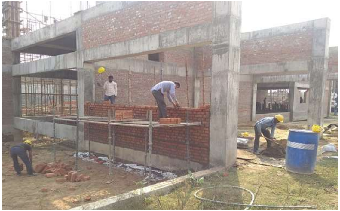
Air Blower Building - DG Partition Brickwork
