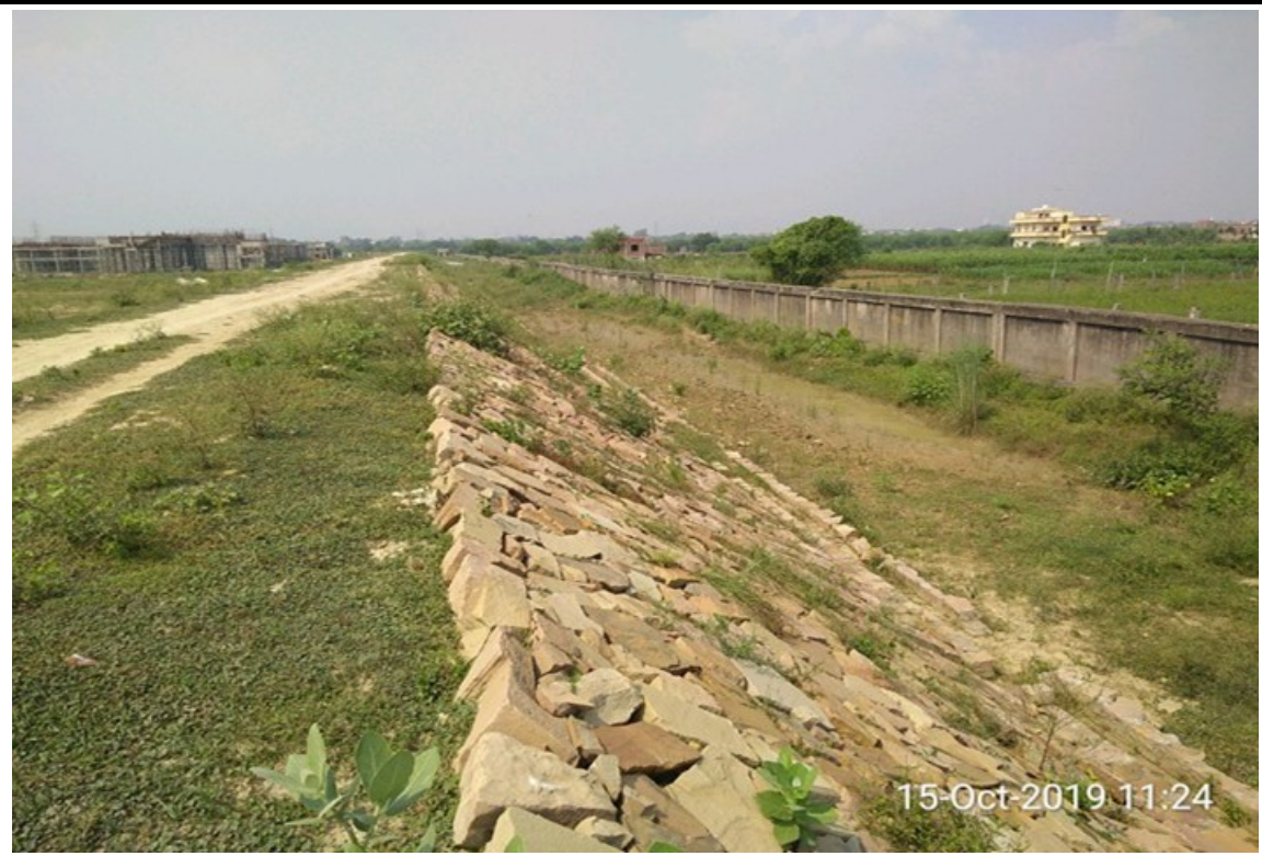
Bund wall - North
