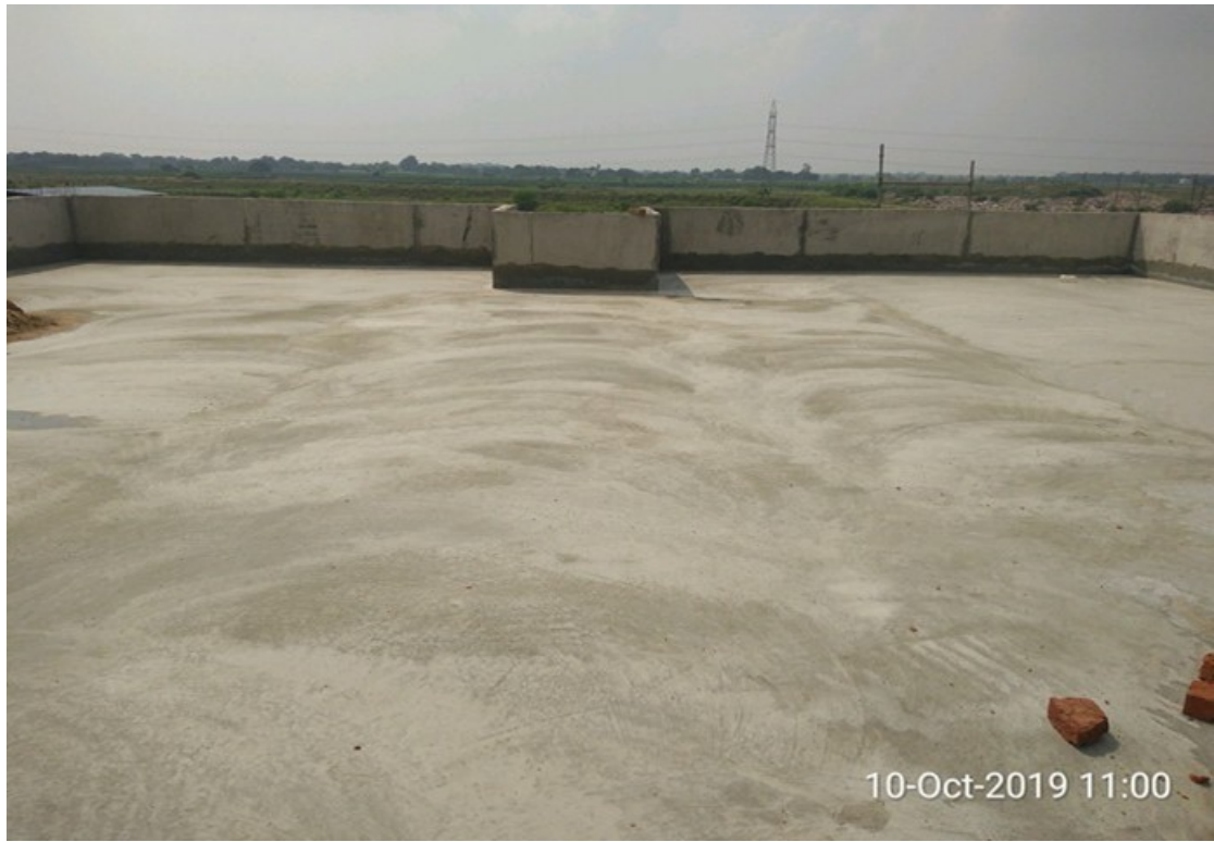
Water proofing at Administrative building
