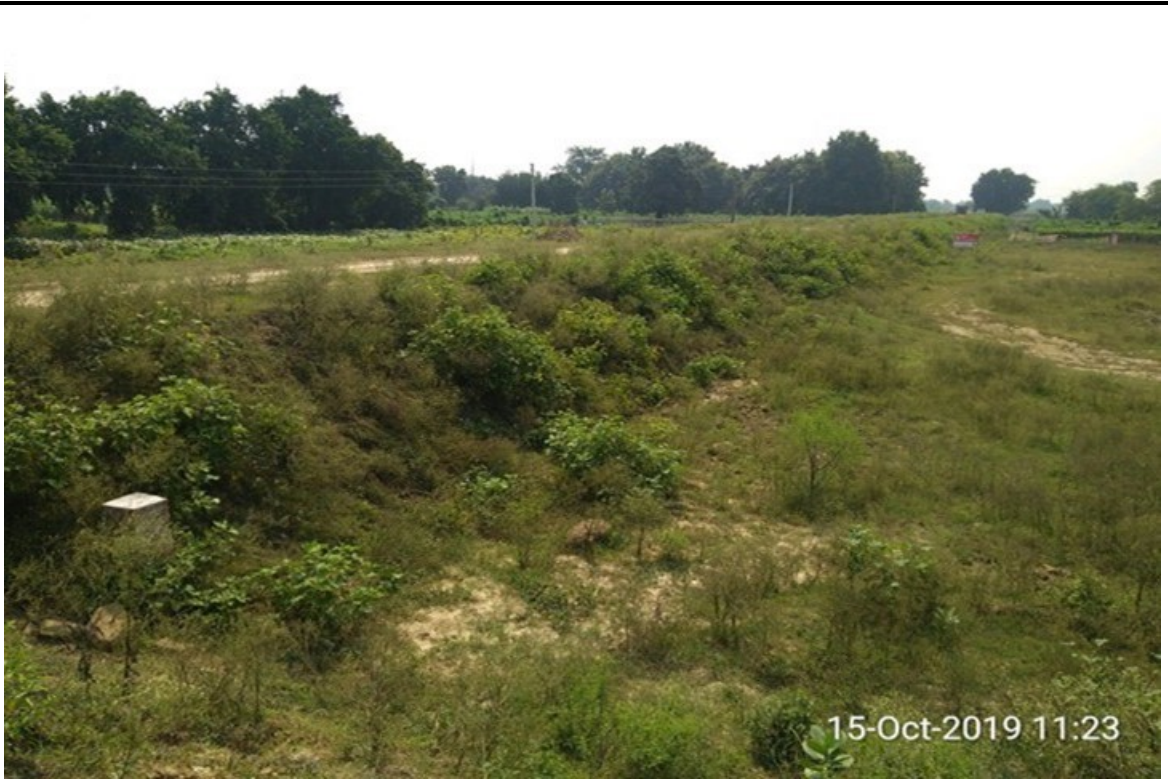
Bund wall - East
