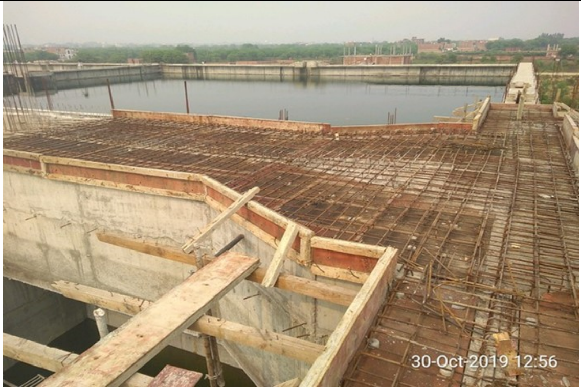
SBR Inlet channel walkway slab
