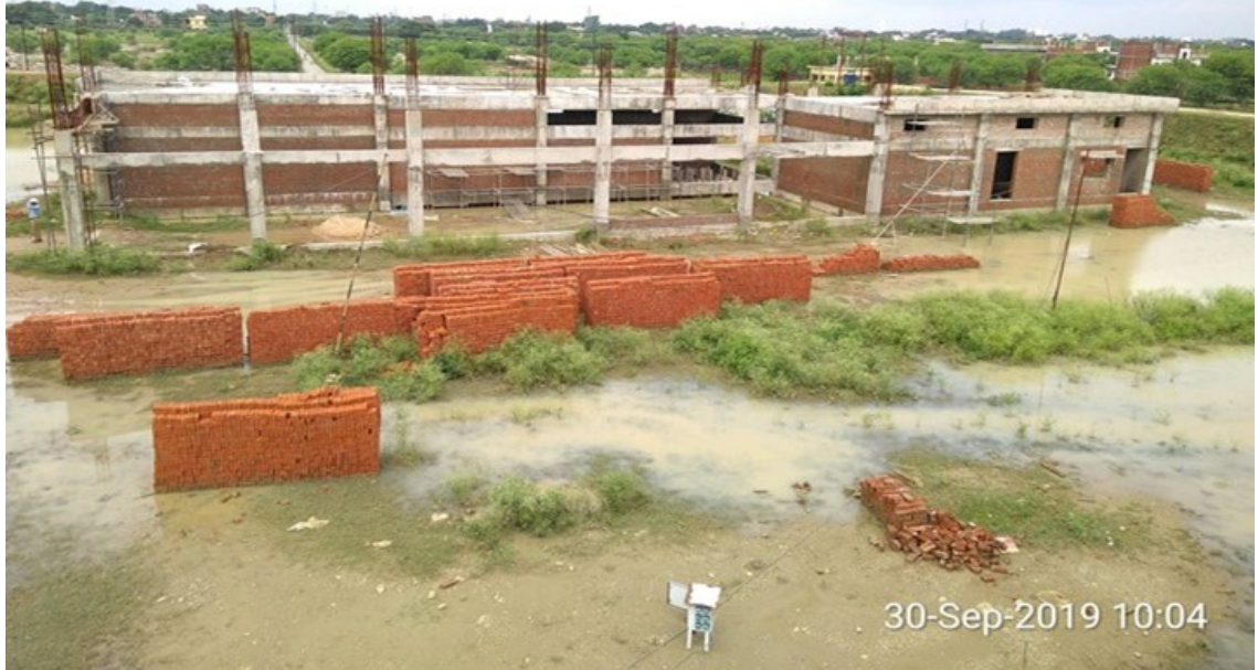
Air Blower & MCC Building
