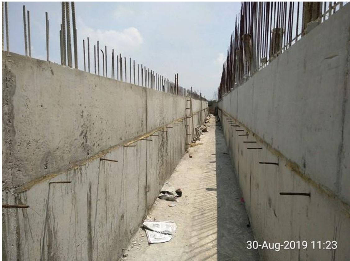
Inlet channel to Basin 1 & 4
