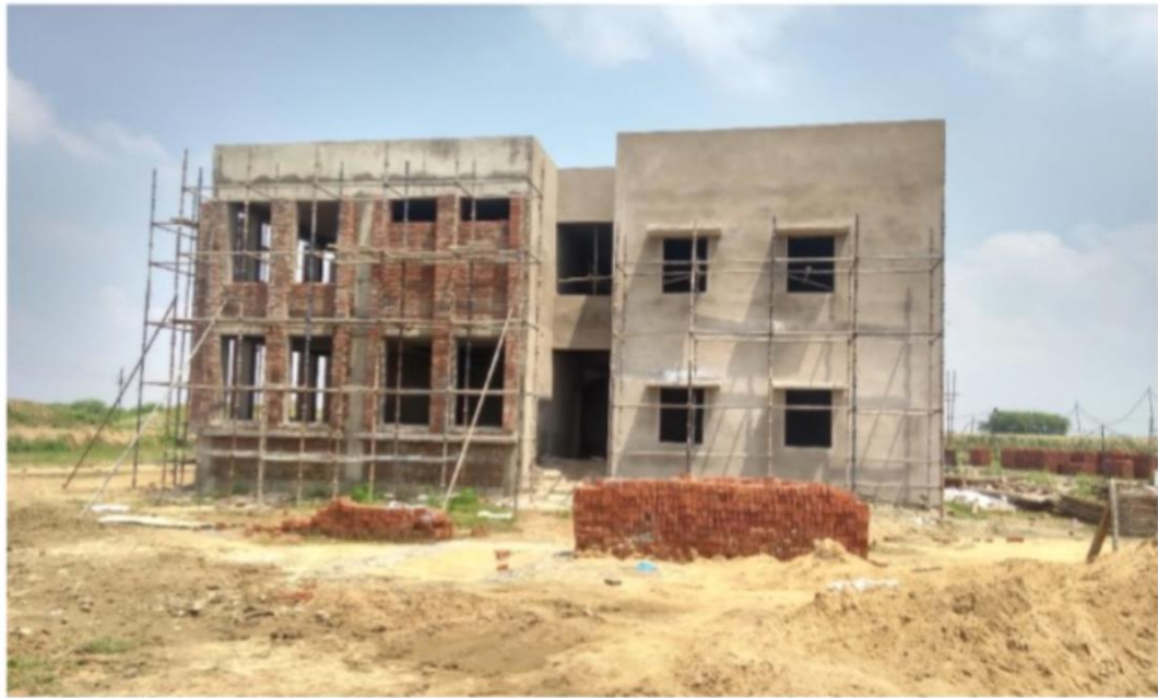
Plastering work – Behind
