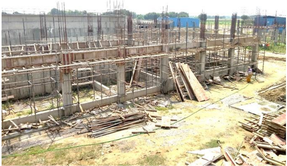
Tie beam work is in progress
