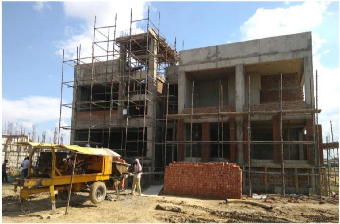
Head room work is in progress
