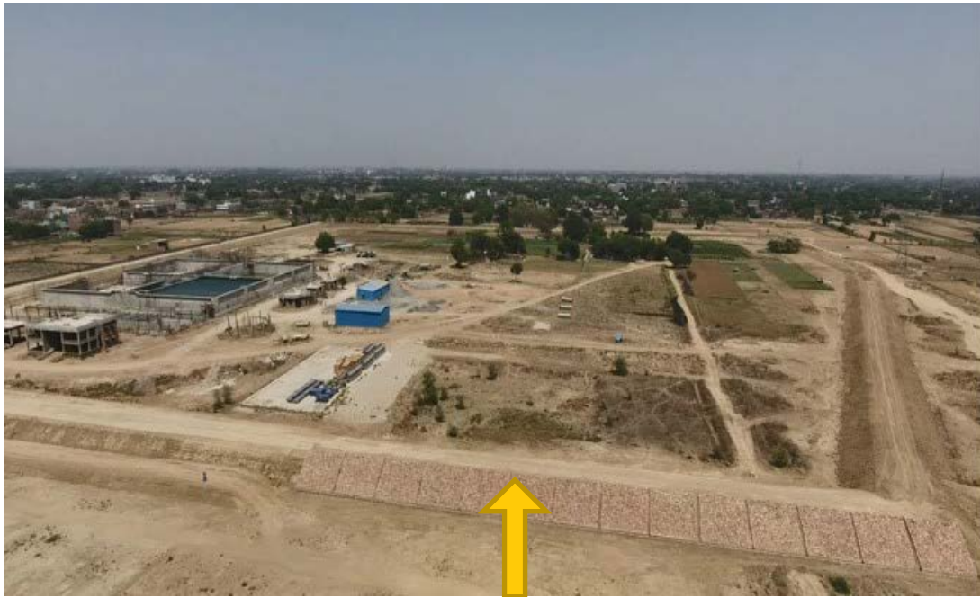
Stone pitching on Northern side
