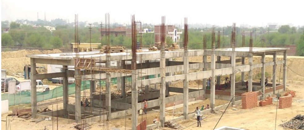
At roof level
