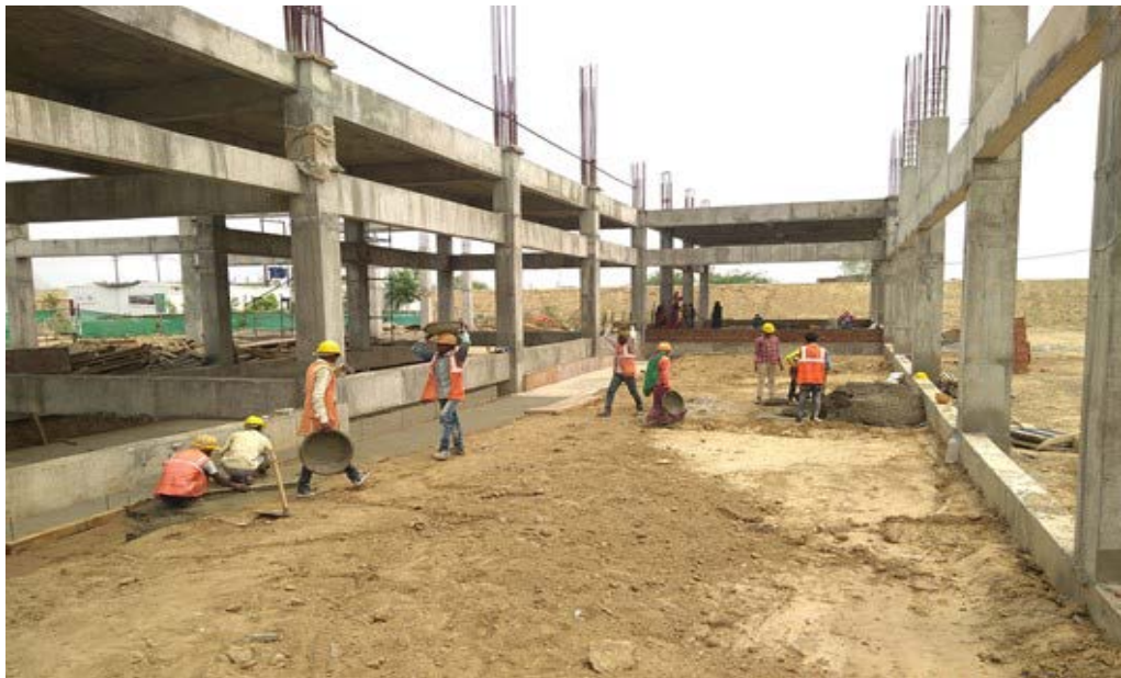
SBR air blower room, HT room, MCC room, Transformer Yard & DG set area
