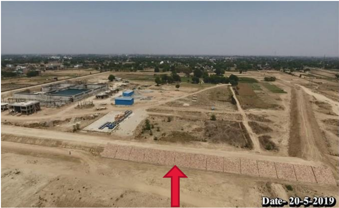
Stone pitching on Northern side
