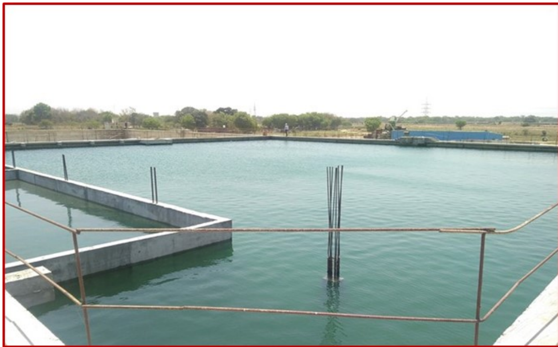
Basin 3 water level 5.4m
