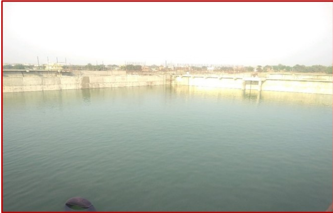
Basin 3 water level 4m
