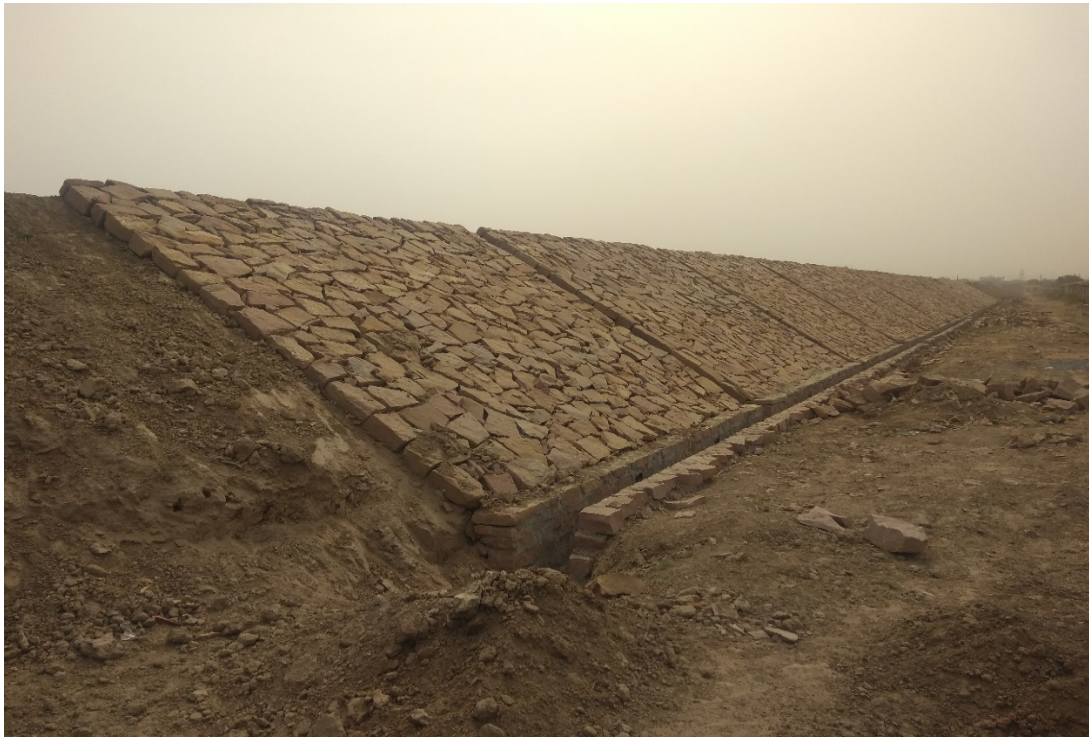
Stone pitching on Northern side
