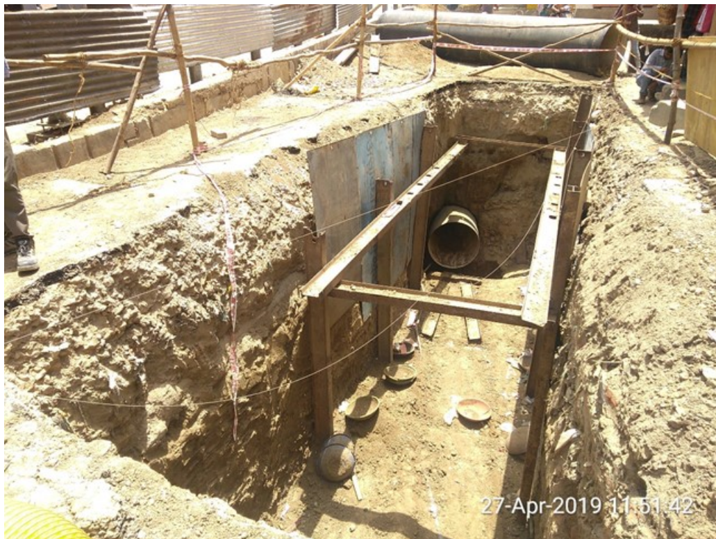
Trenchless M.S. Pipe laying
