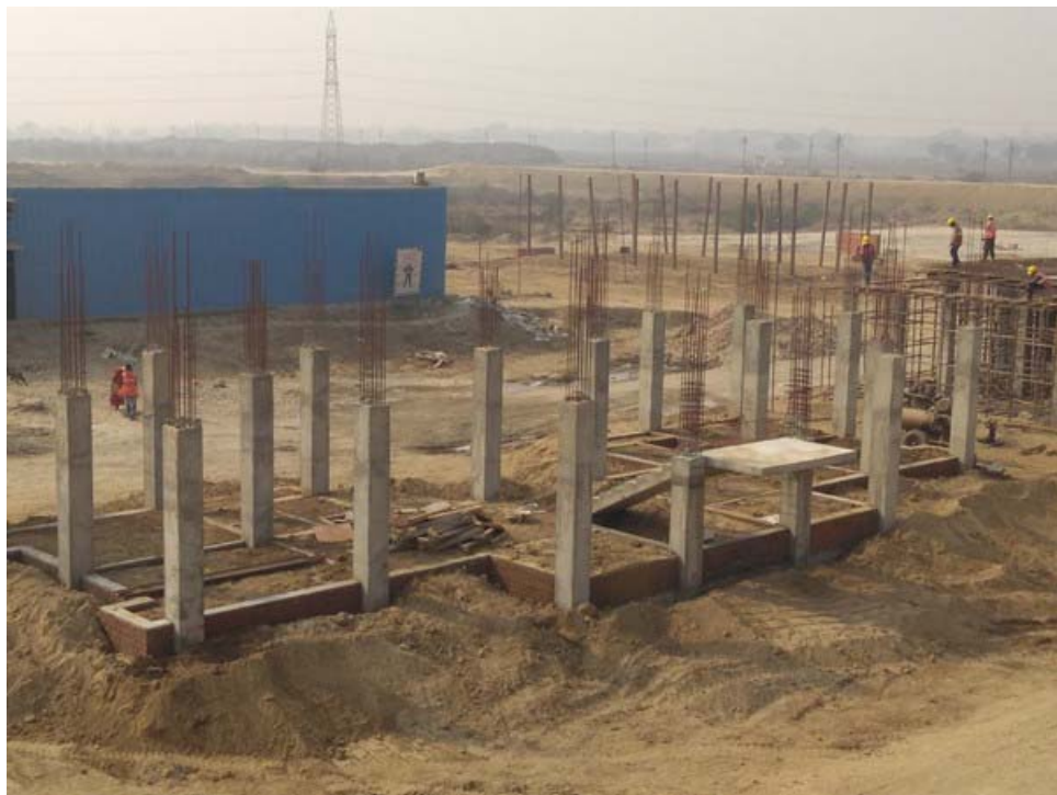
Type – 2 ( Column concrete )
