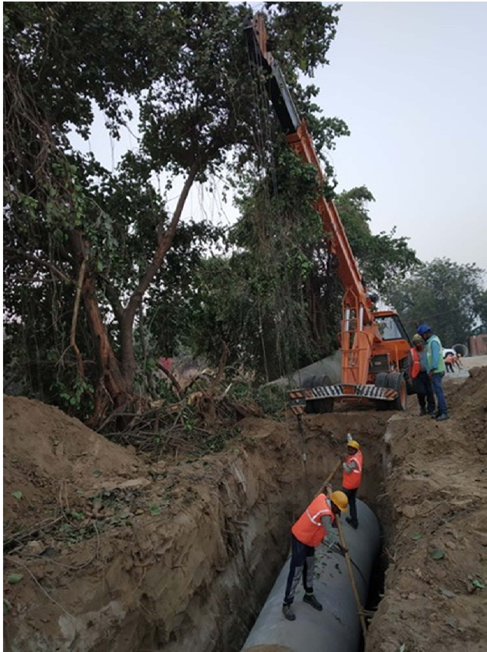
PSC Pipe laying
