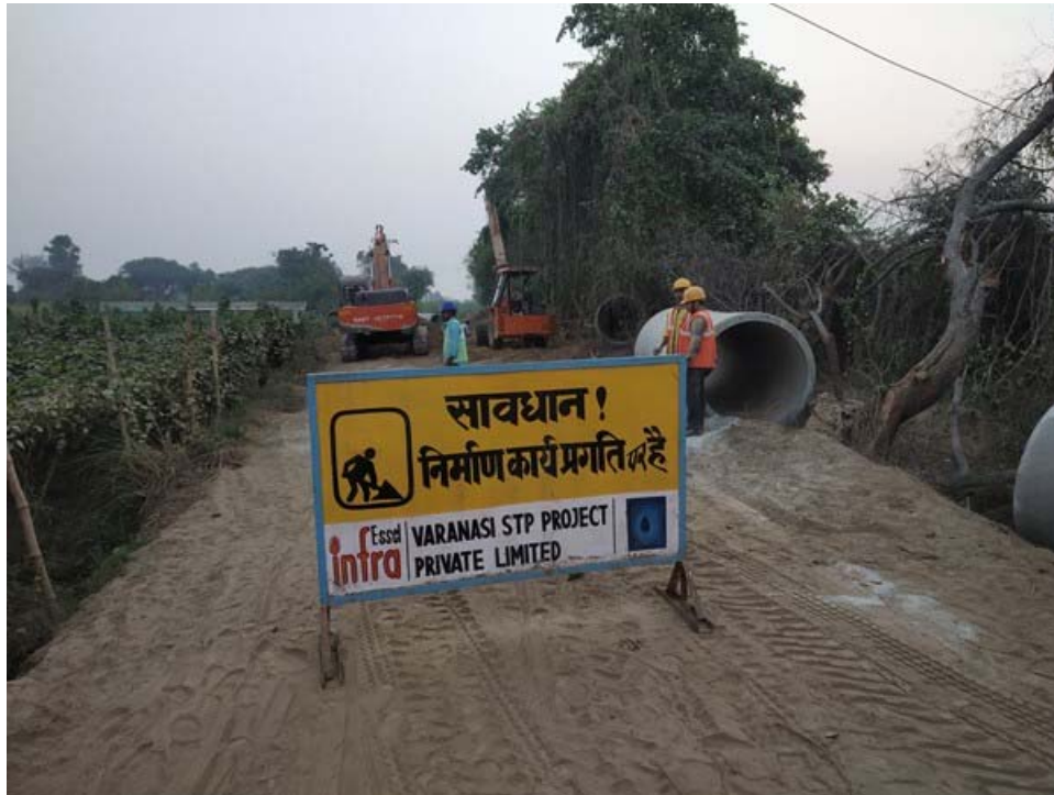
PSC Pipe laying
