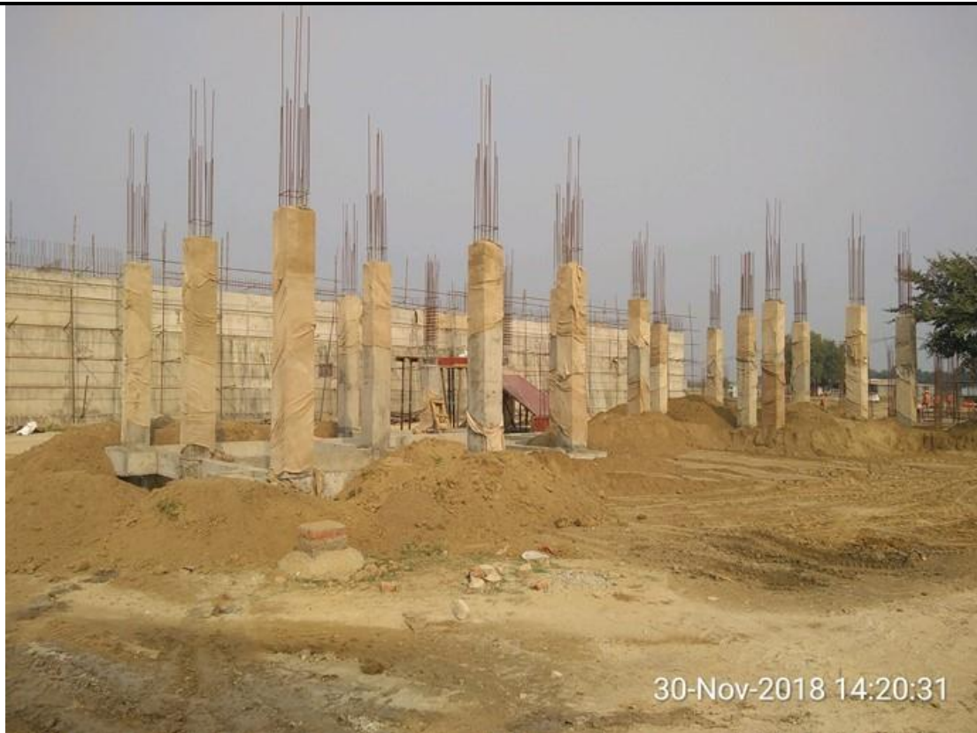
Type – 2 ( Column concrete )
