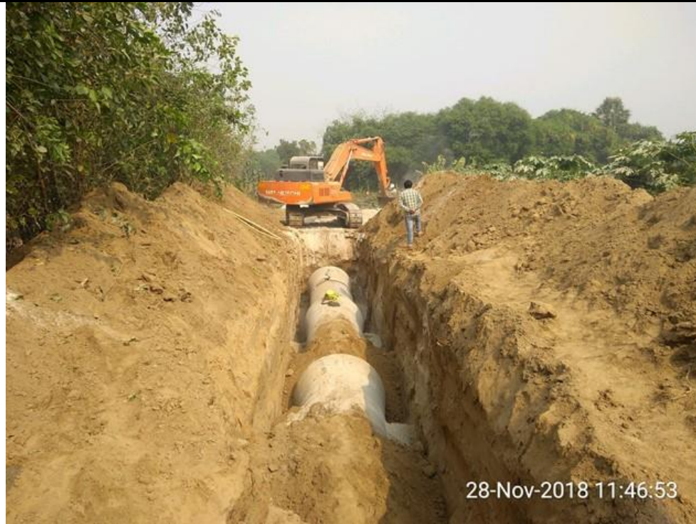
PSC Pipe laying
