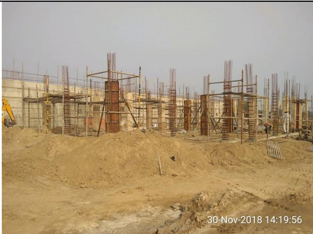
Type – 4 ( Column concrete )
