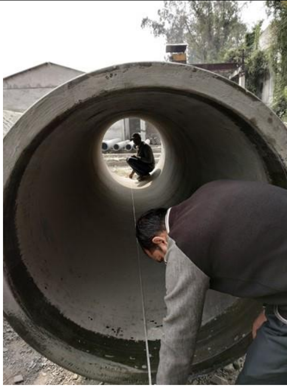
Length dimension checking
