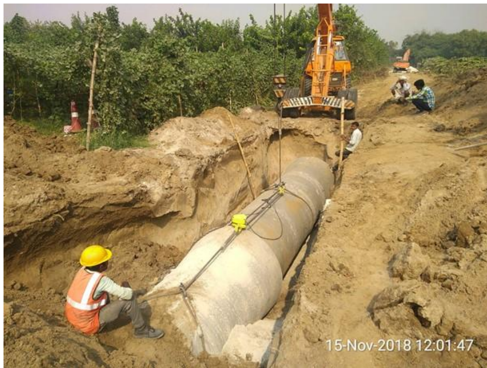
PSC Pipe laying
