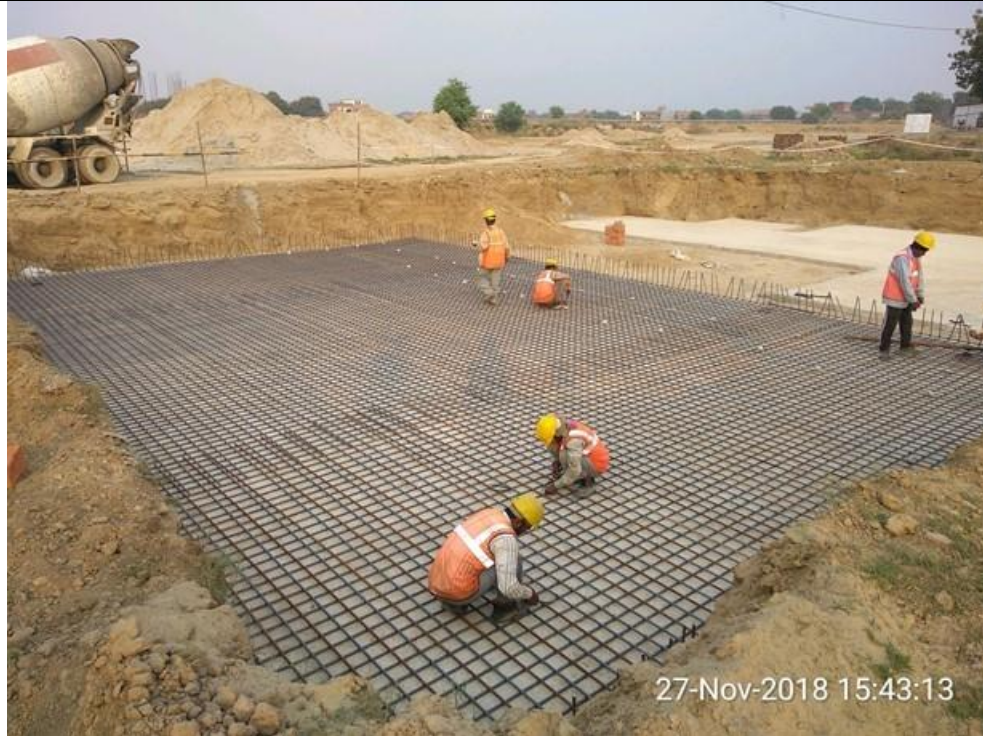
Reinforcement for footing
