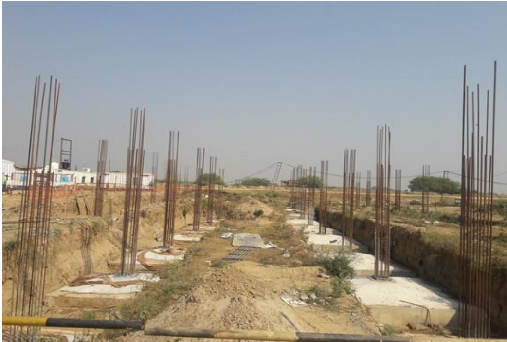
Footing reinforcement
