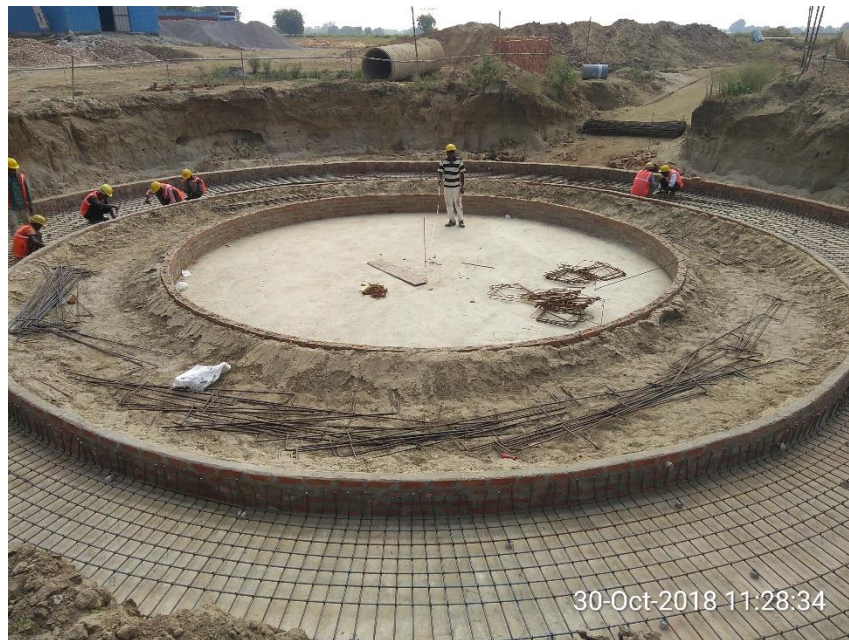
Footing reinforcement
