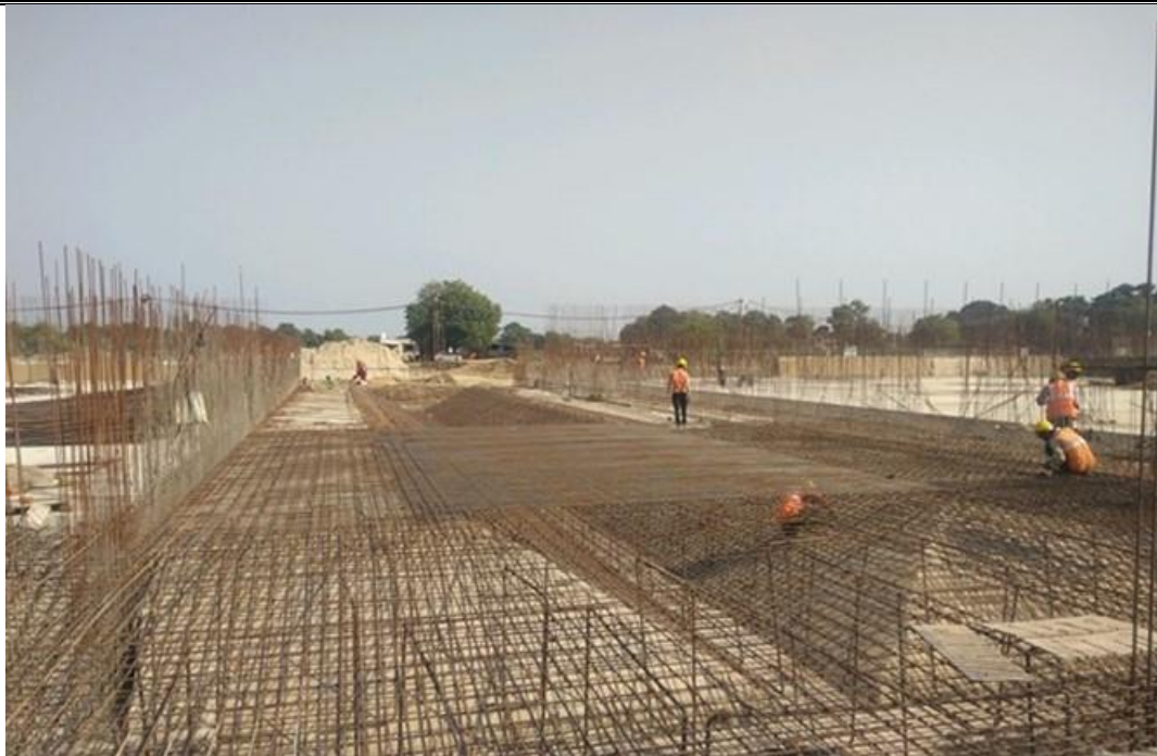
Reinforcement work
