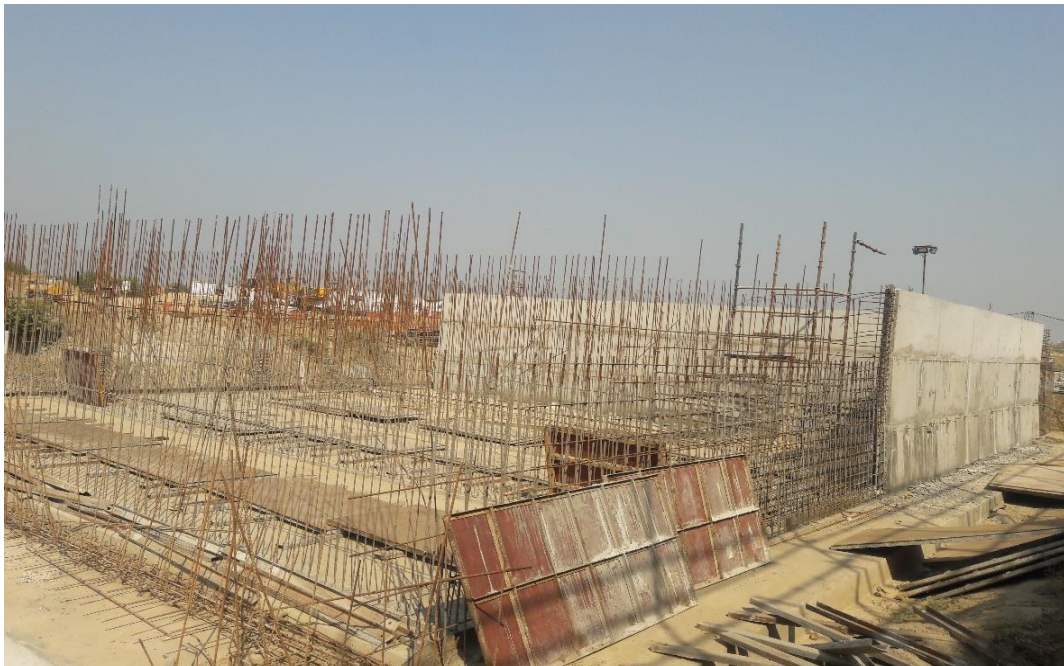
Shuttering for wall
