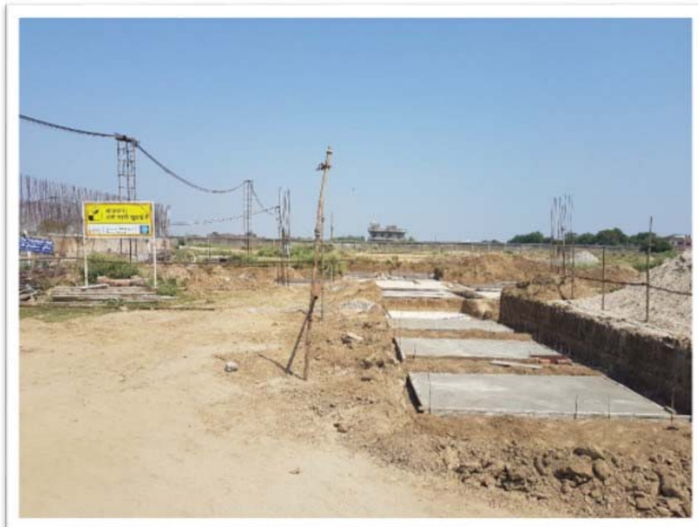
Footing PCC work
