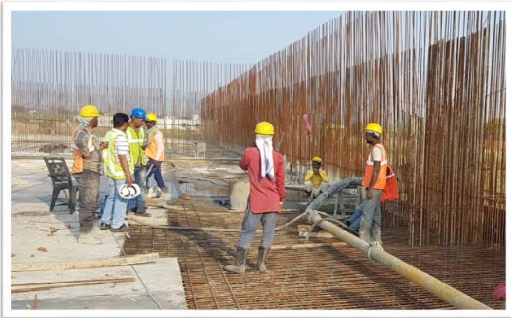
RCC Footing Concrete
