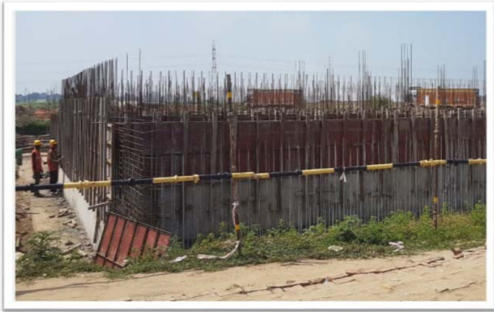
Shuttering for wall
