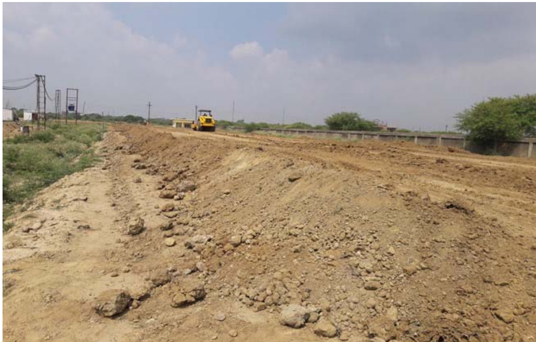
Soil filling and Compaction
