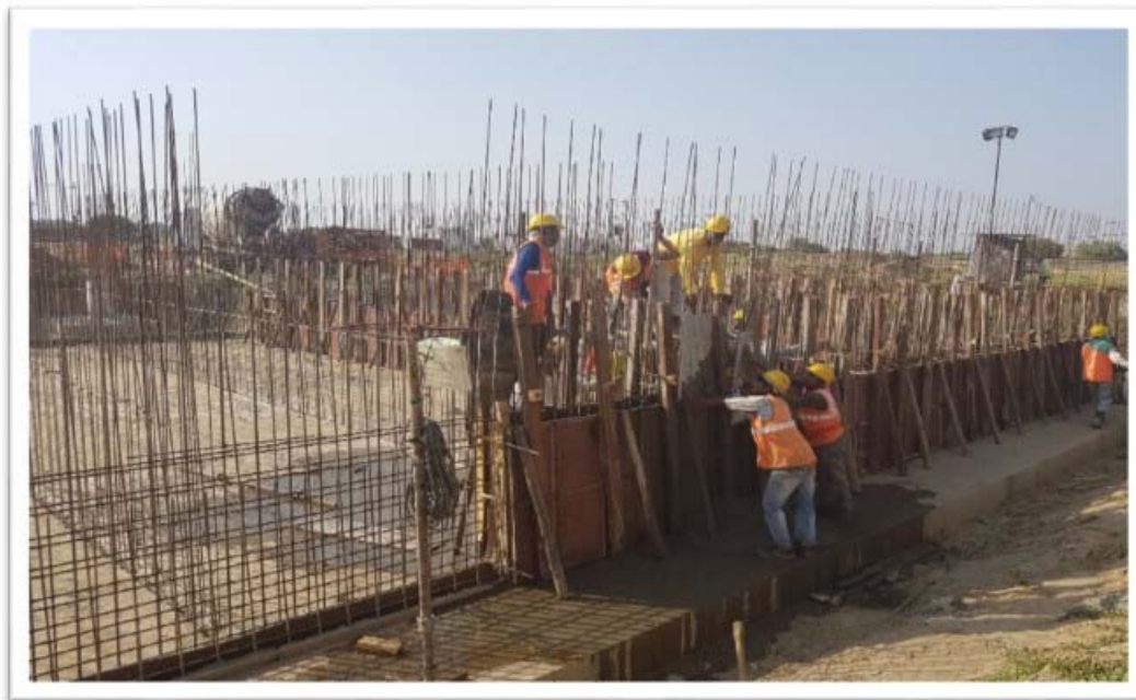
Side wall Concreting work
