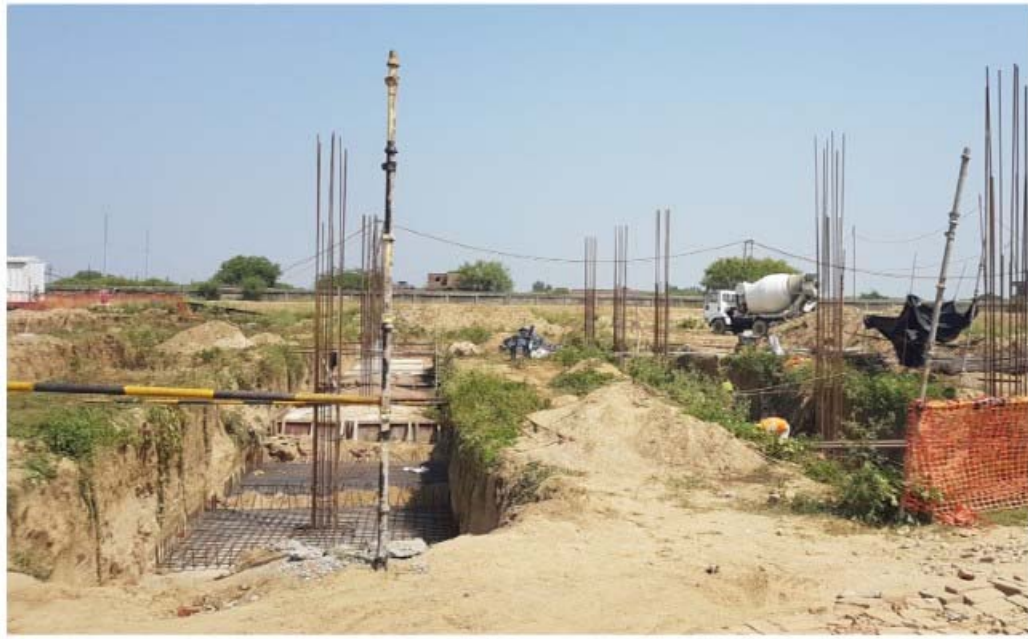
Footing reinforcement
