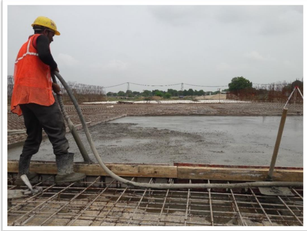
RCC Footing Concrete
