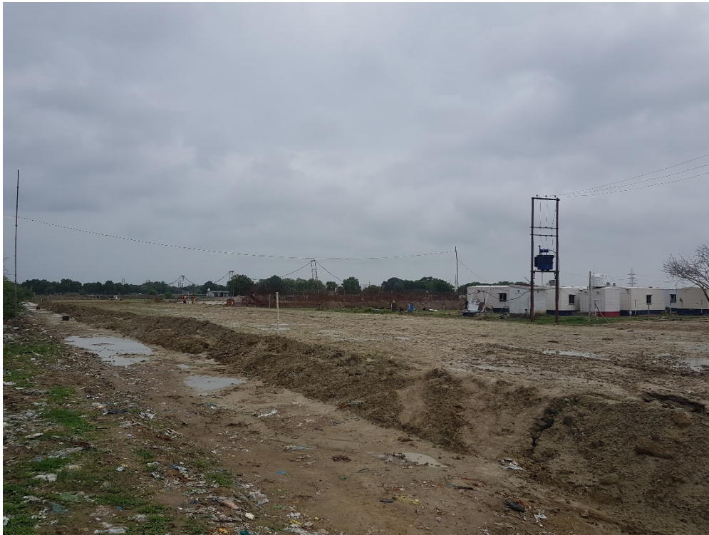
North side view
