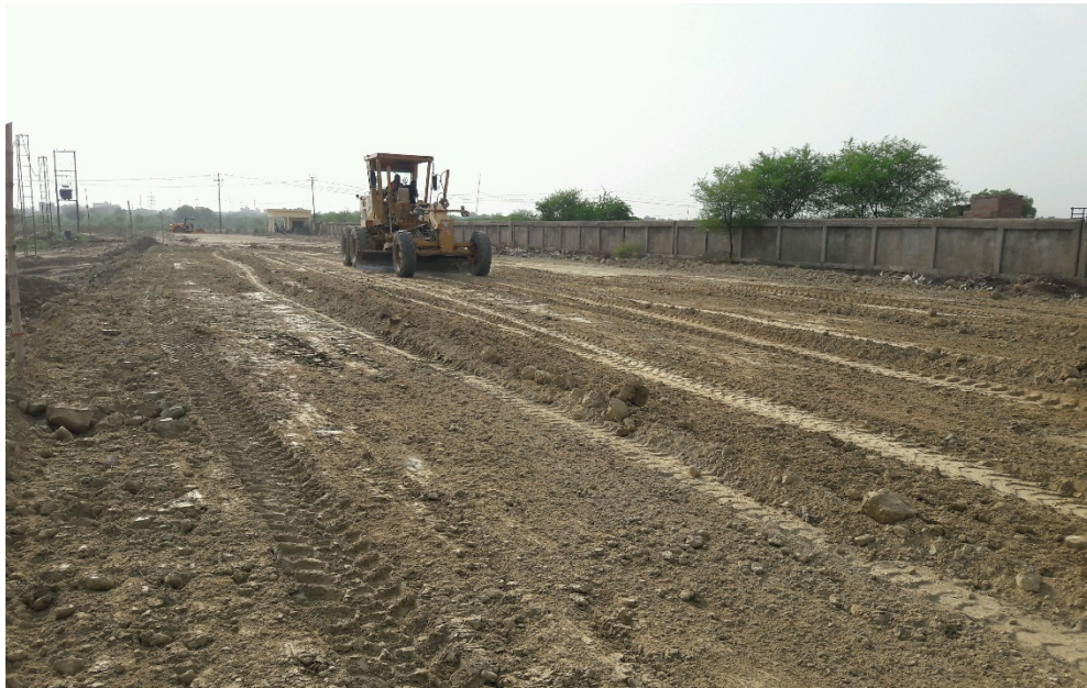
Levelling and compaction
