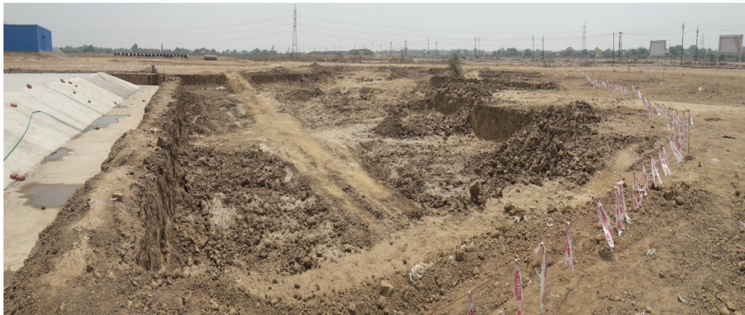
Earth work excavation
