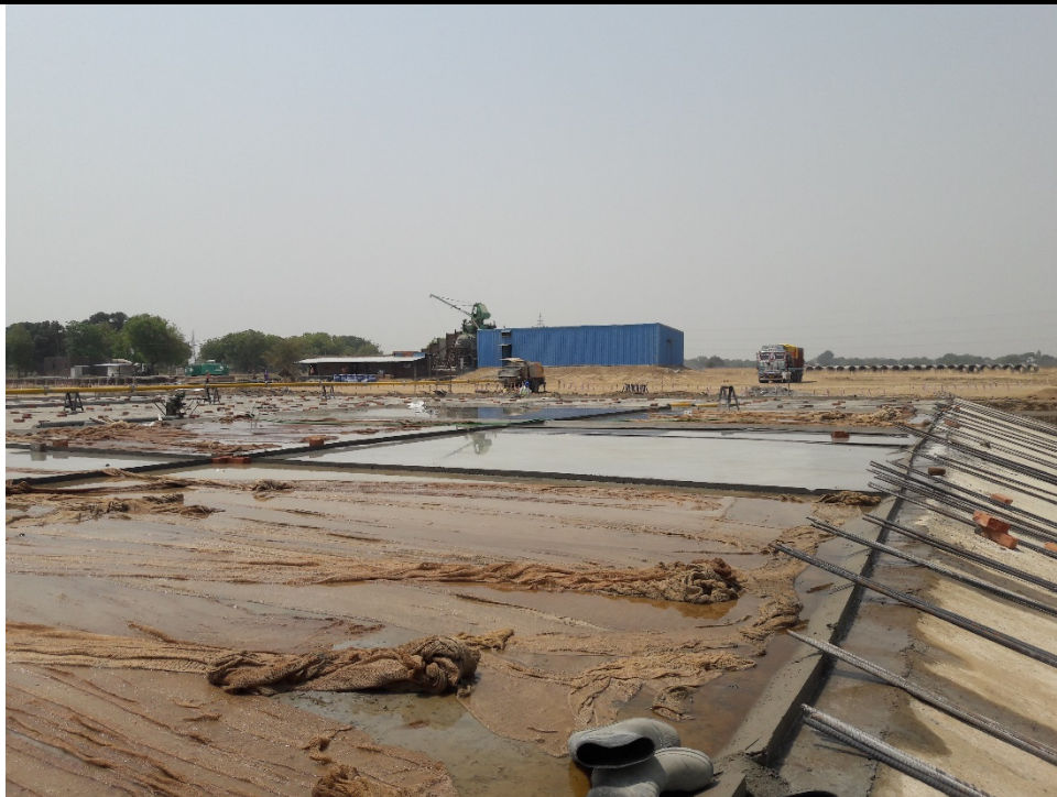
Curing for PCC
