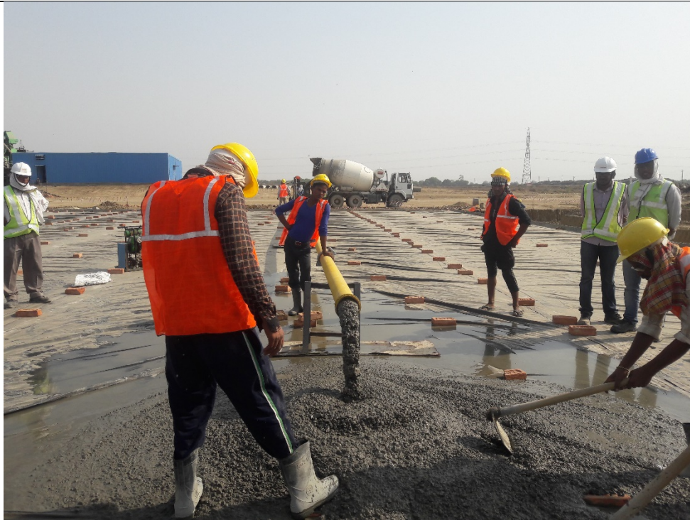
PCC being laid
