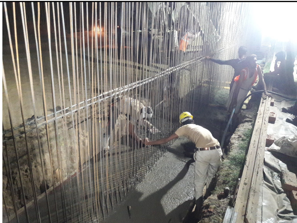
Raft concrete laying
