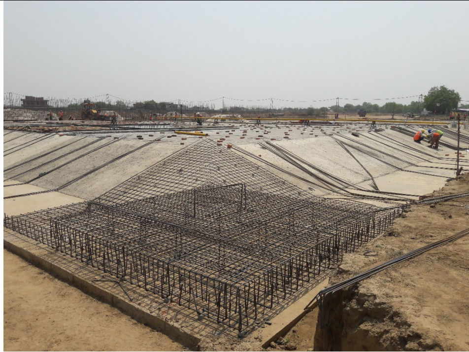
Steel reinforcement for footing
