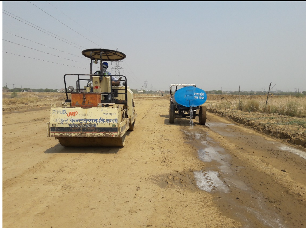
Levelling and compaction
