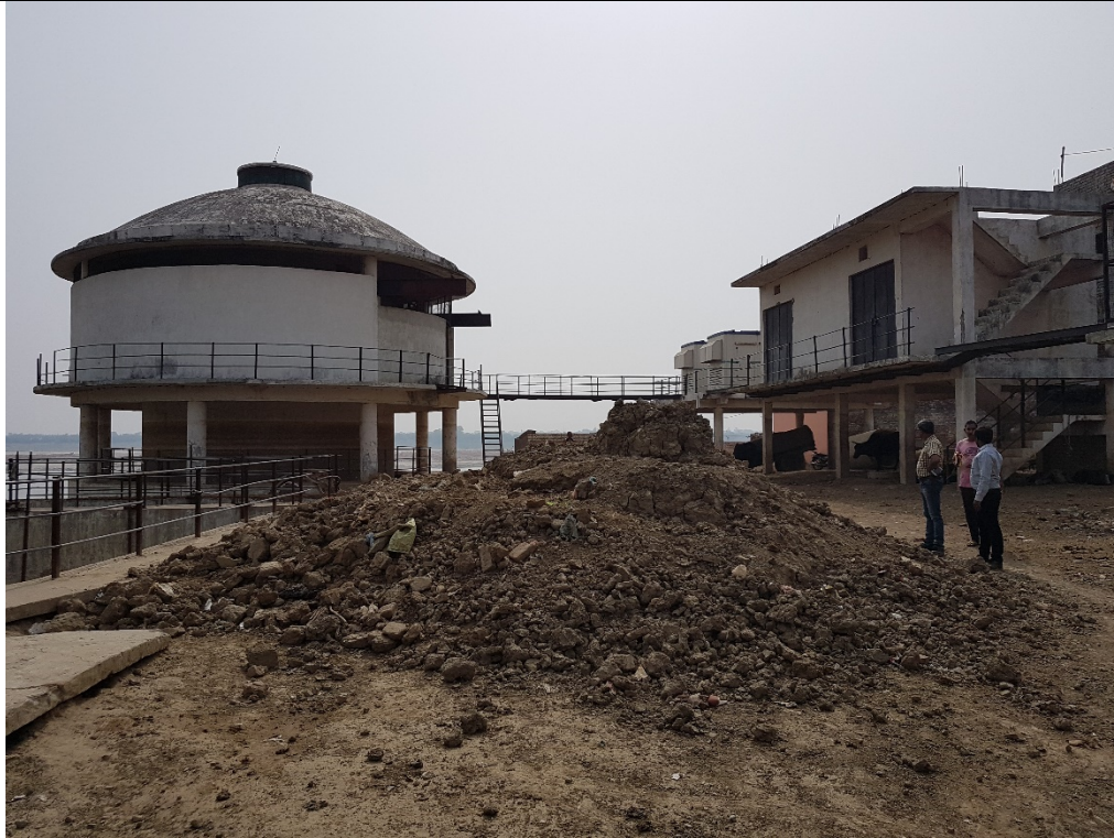
Desilting inlet chamber
