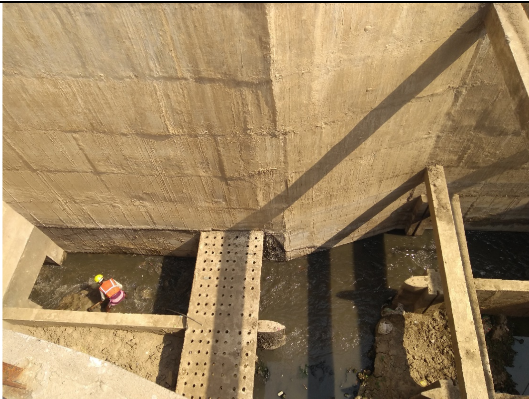
Desilting Inlet chamber
