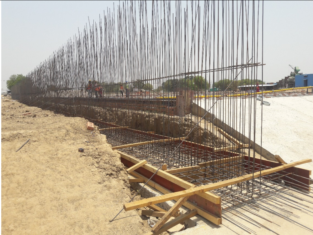
Steel reinforcement for wall
