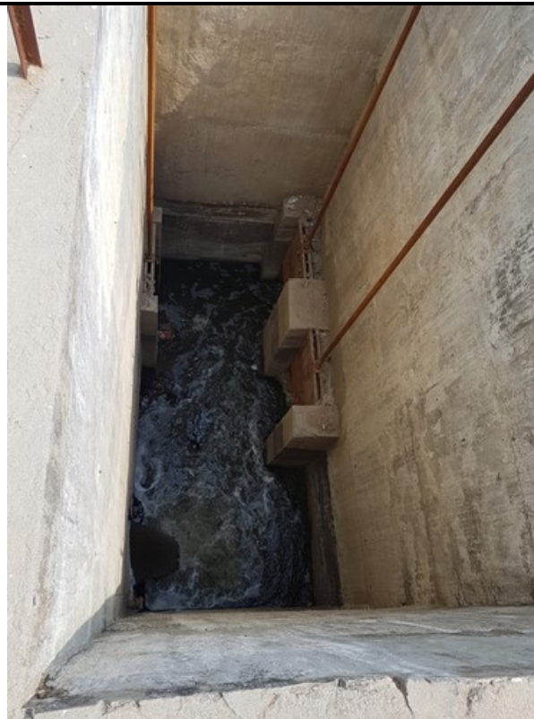
Desilting Inlet chamber
