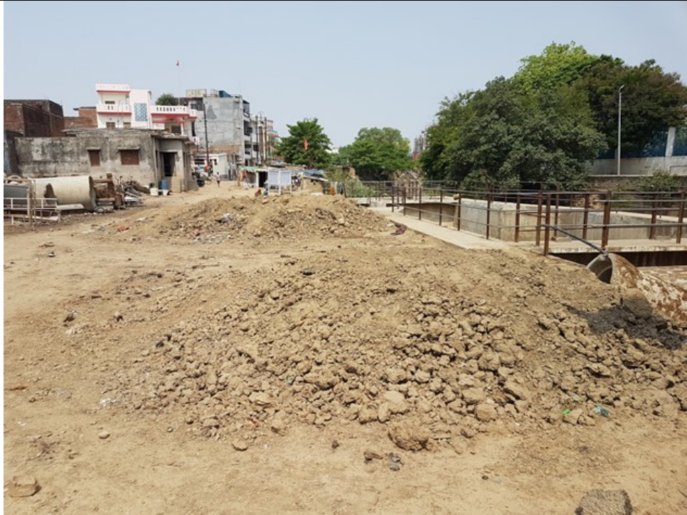
Desilting inlet chamber
