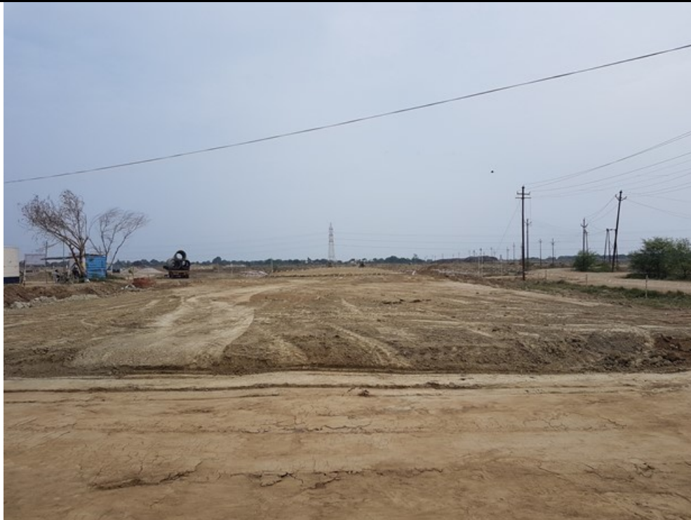
Levelling and compaction
