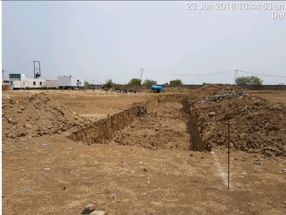
Earth work excavation
