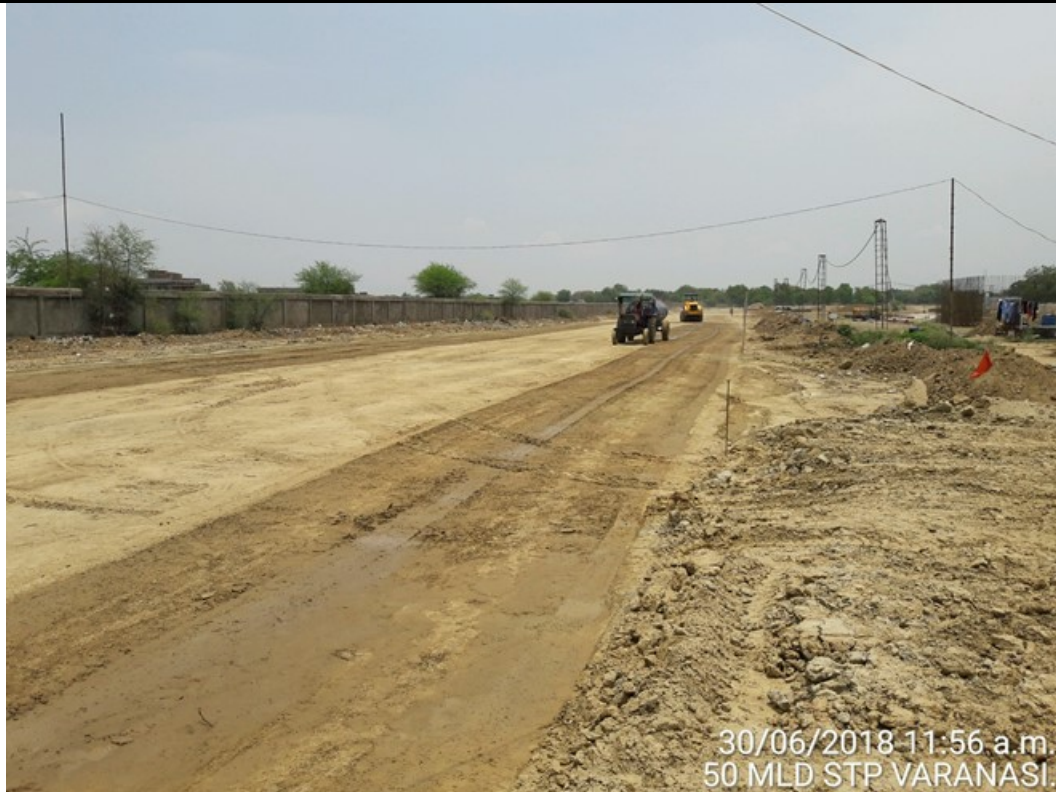
Levelling and compaction
