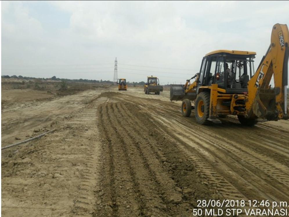
Levelling and compaction
