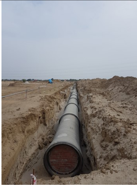
PSC Pipe laying
