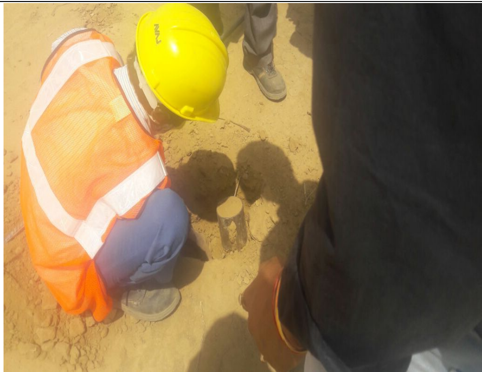
Compaction test being done at site
