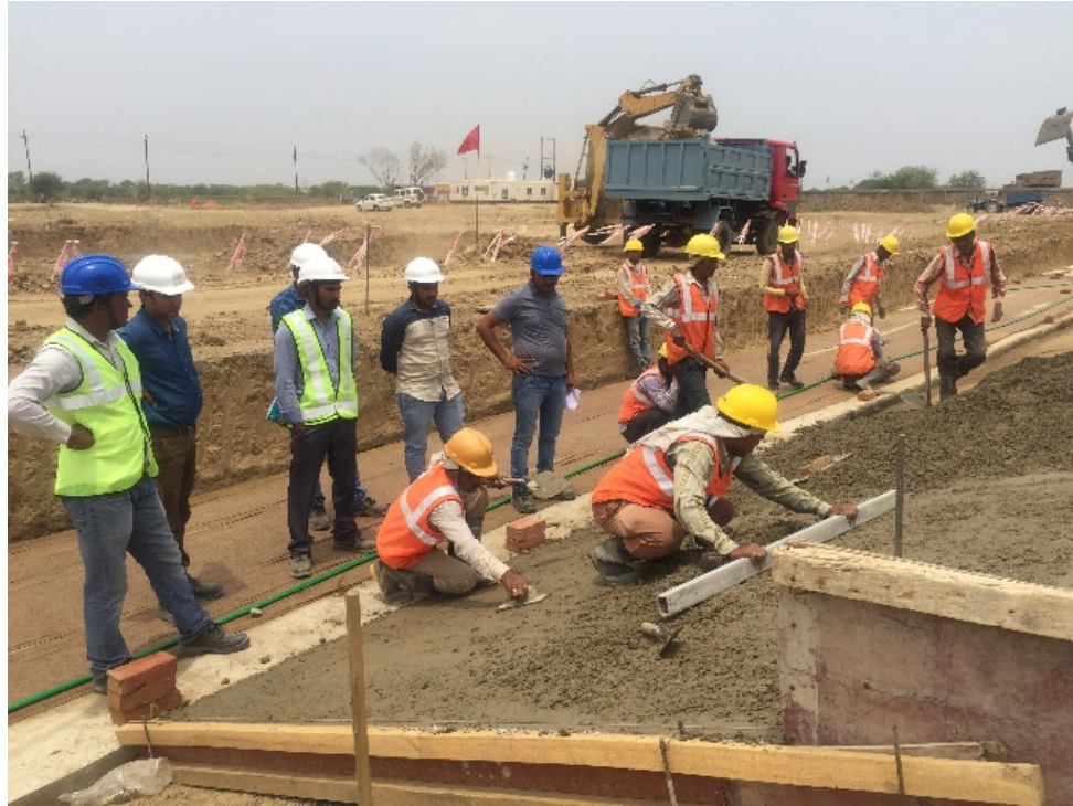
PCC concrete laying
