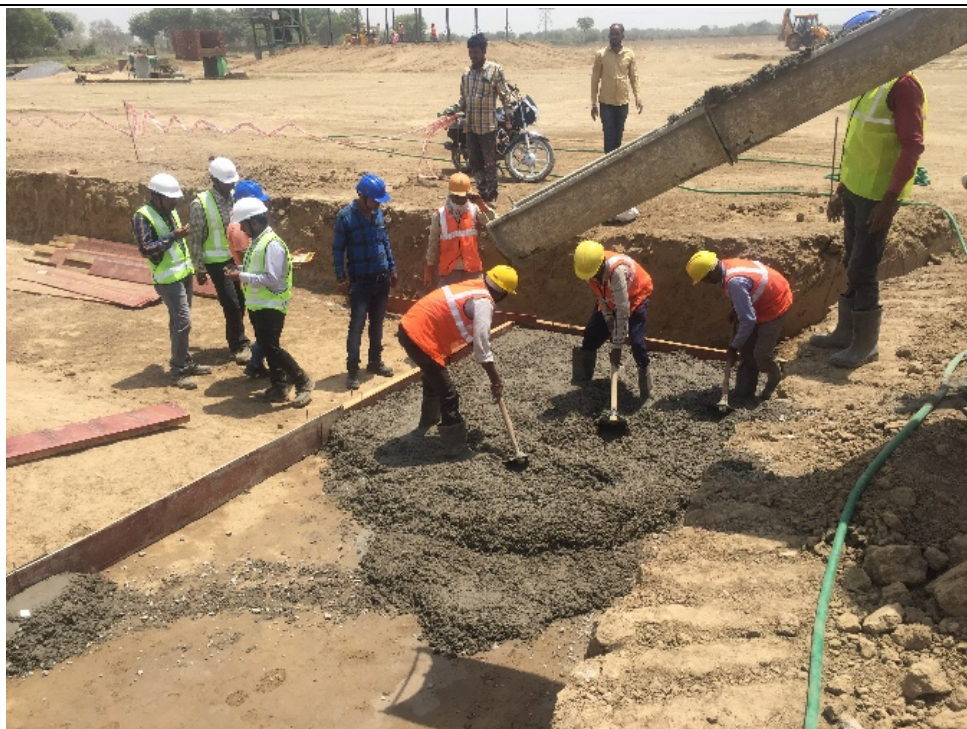
PCC being laid
