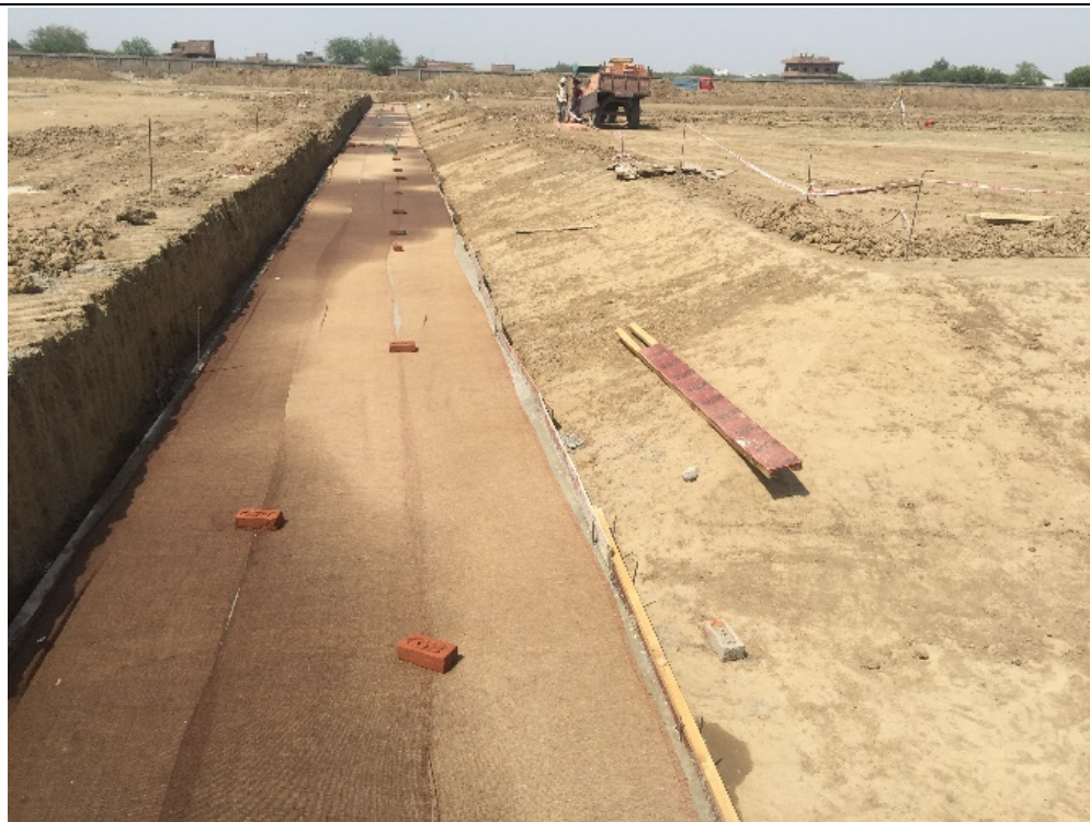
Curing for PCC
